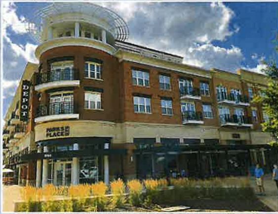
Figure 40: Developments in the Nickel Plate District
