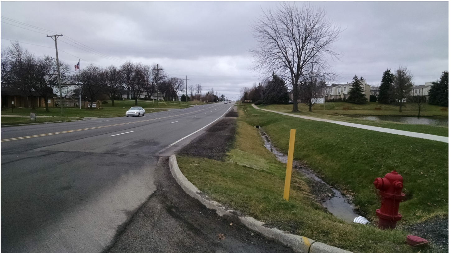
Looking south along road widening and gravel shoulders
