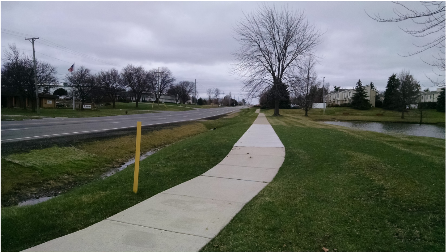
Looking south along sidewalk and ditch line improvements
