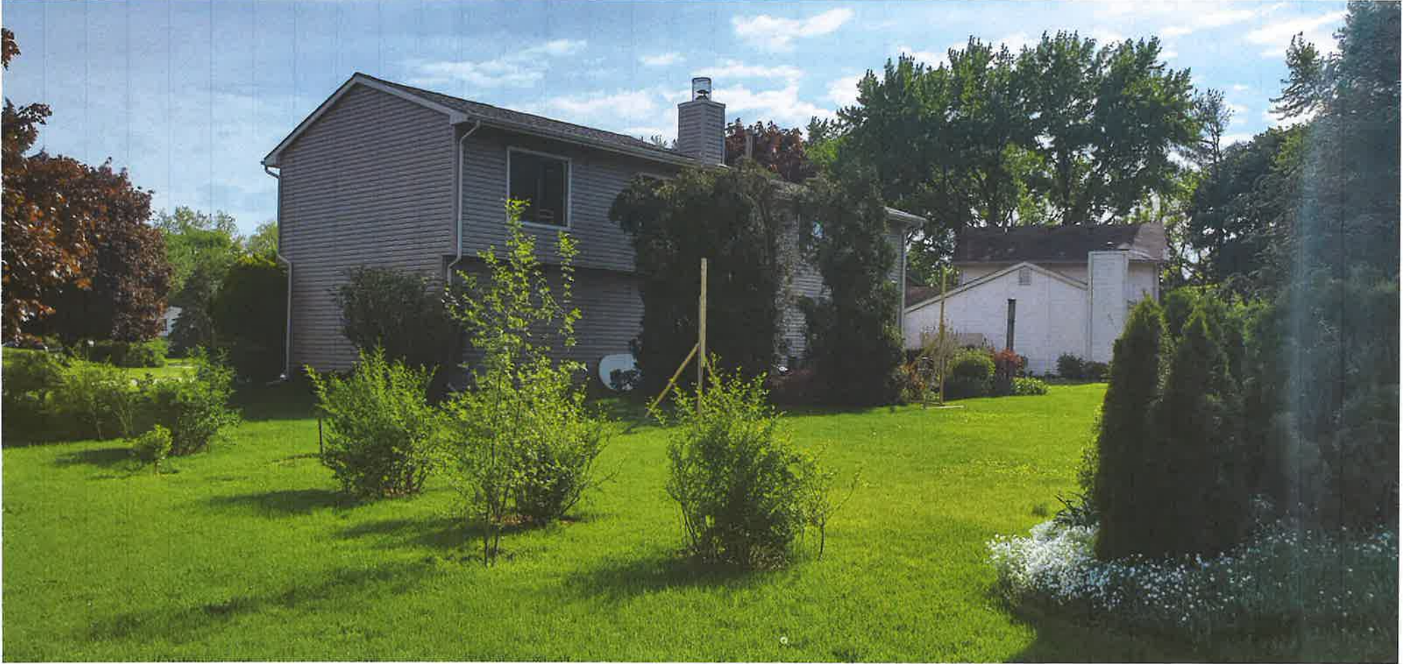
VIEW OF REAR FROM CRAWBROOKE
