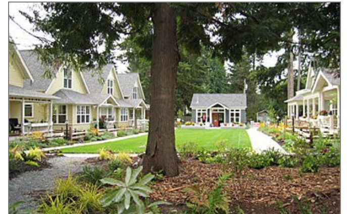
Source: Cottage Company
