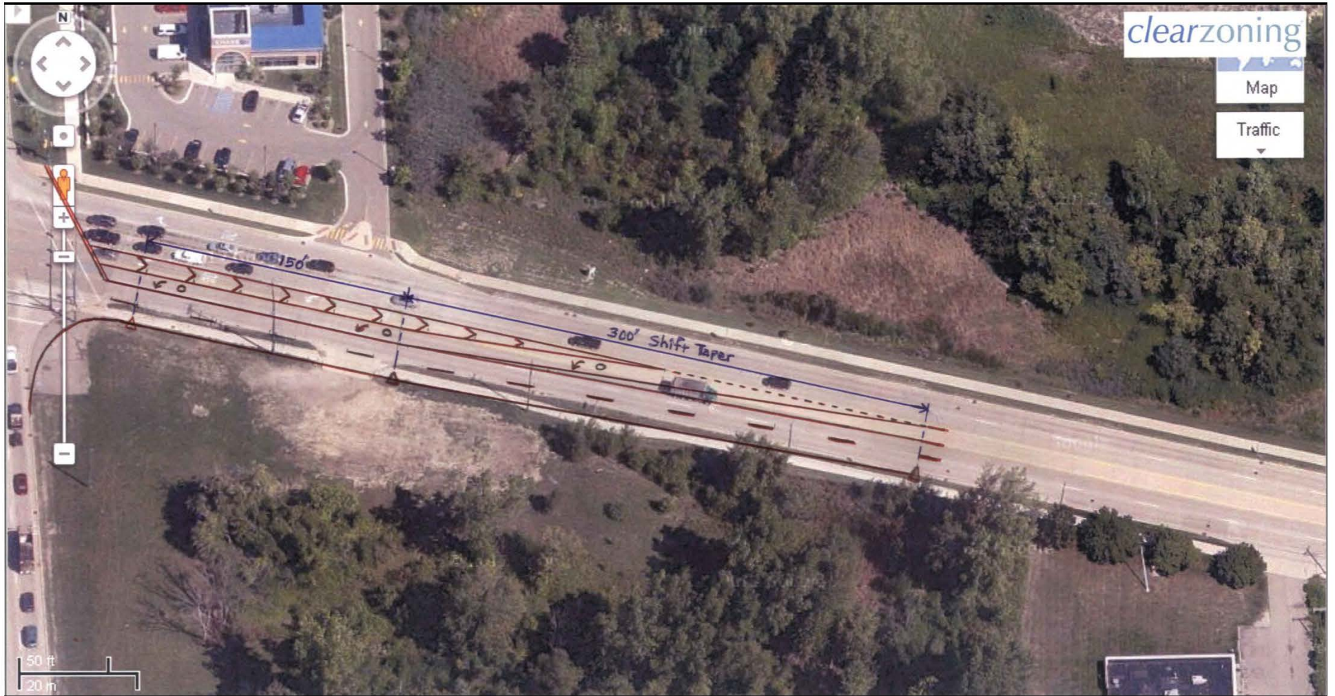
Figure 2. Widening of East Leg of Intersection
