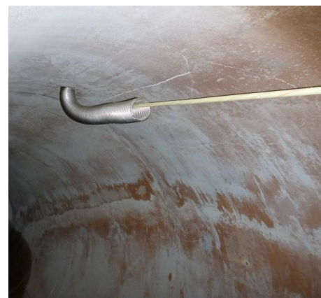
Cable protection into pipe
