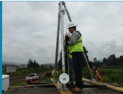
Feeding cable into the pipeline
