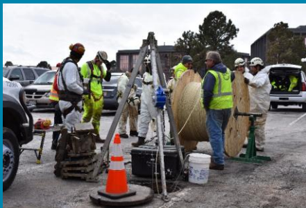
Cable installation staging
