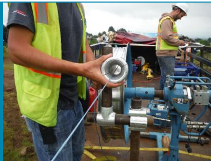
Capstan winch pulling string/cable
