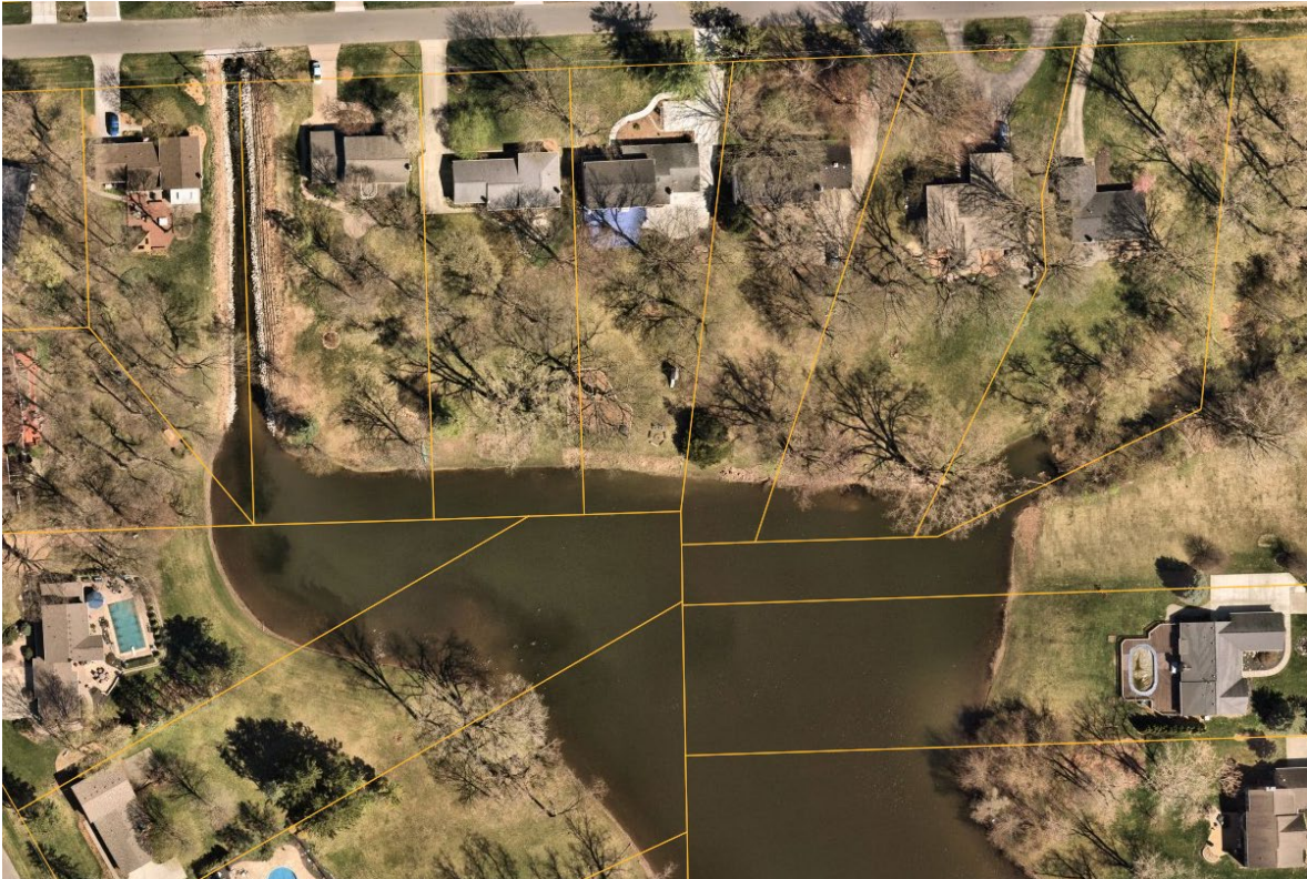
Post-construction aerial photo of Middle Rouge River and Ingersol Creek inlets (April 17, 2025)
