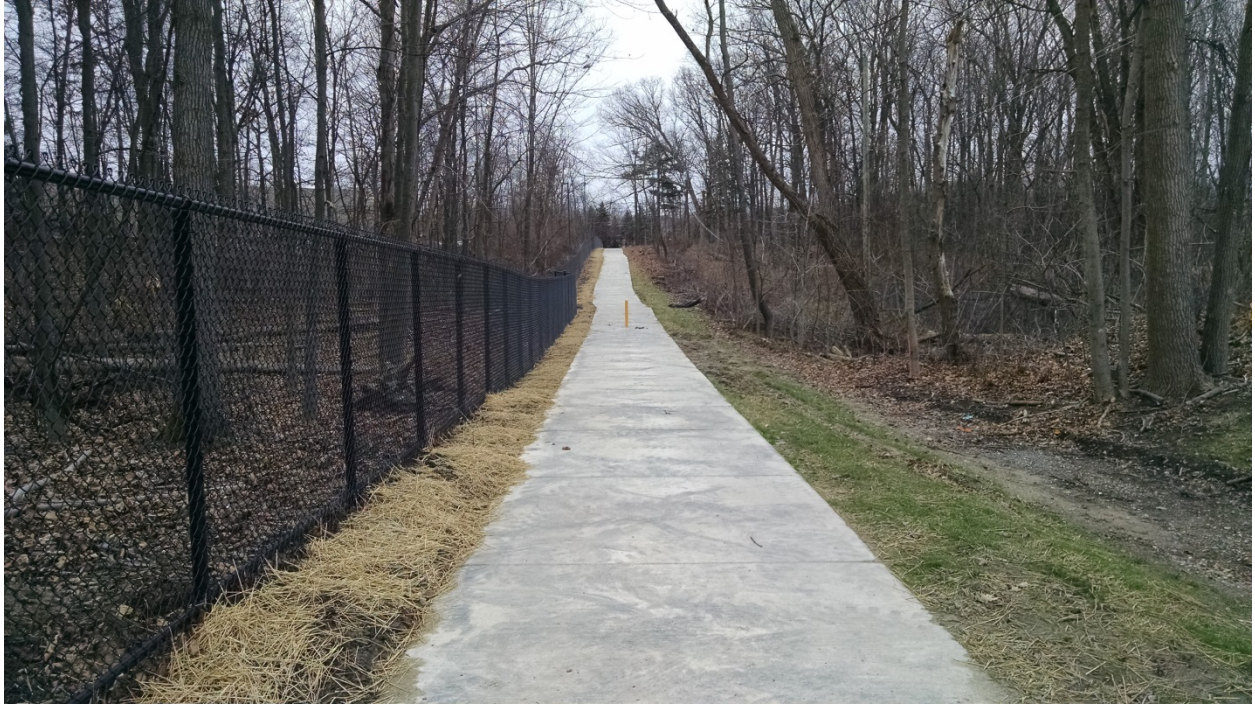
End of roadway, looking east along new path towards Novi Road
