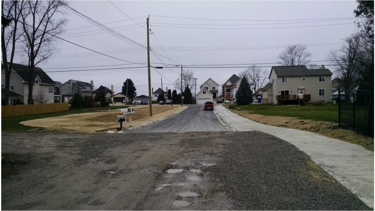
New asphalt roadway and path, looking west towards East Lake Drive
