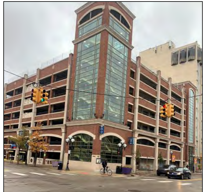
Figure E25: Parking structure with screening and high quality material in Ann Arbor
