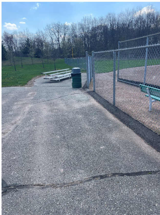
Before: Paved pedestrian and bleacher area
