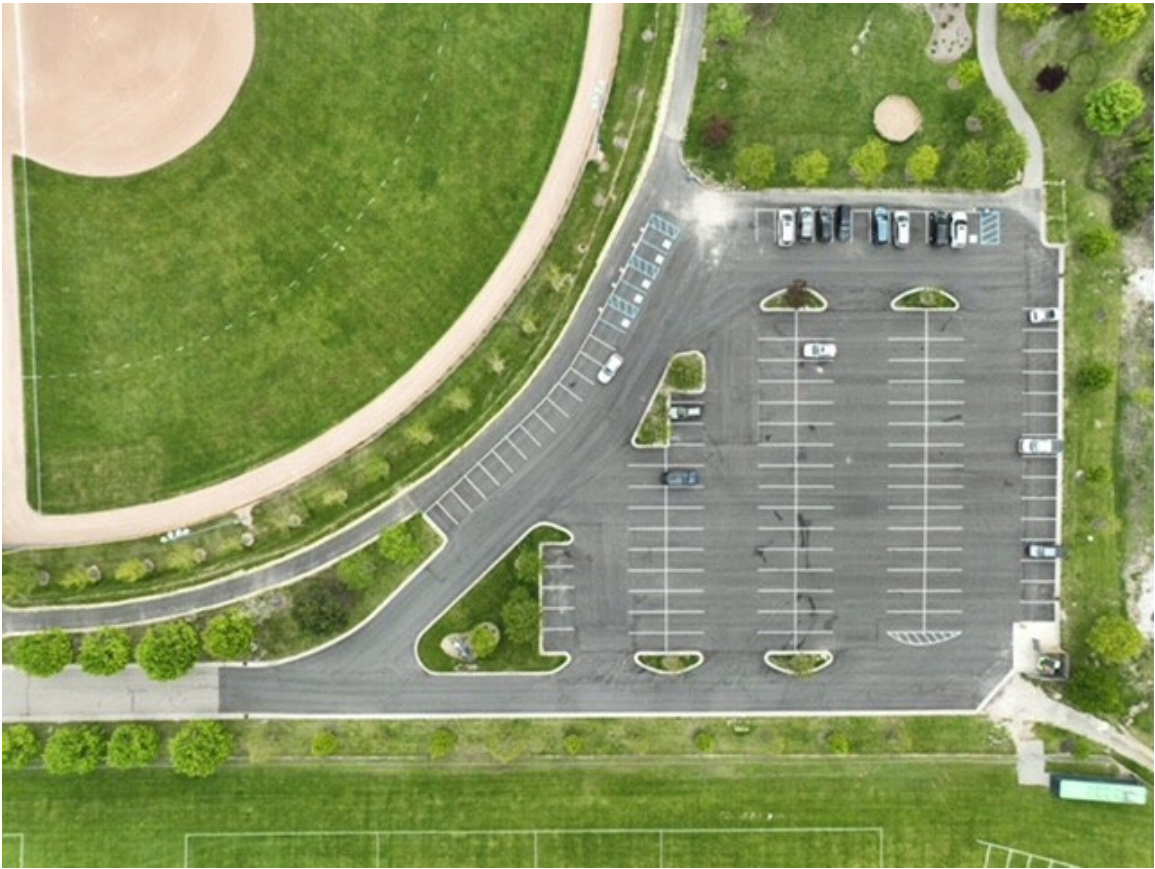
After: Overhead image of parking lot
