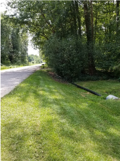
Piping along Garfield Road
