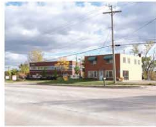
10 The corridor lacks unifying characteristics
