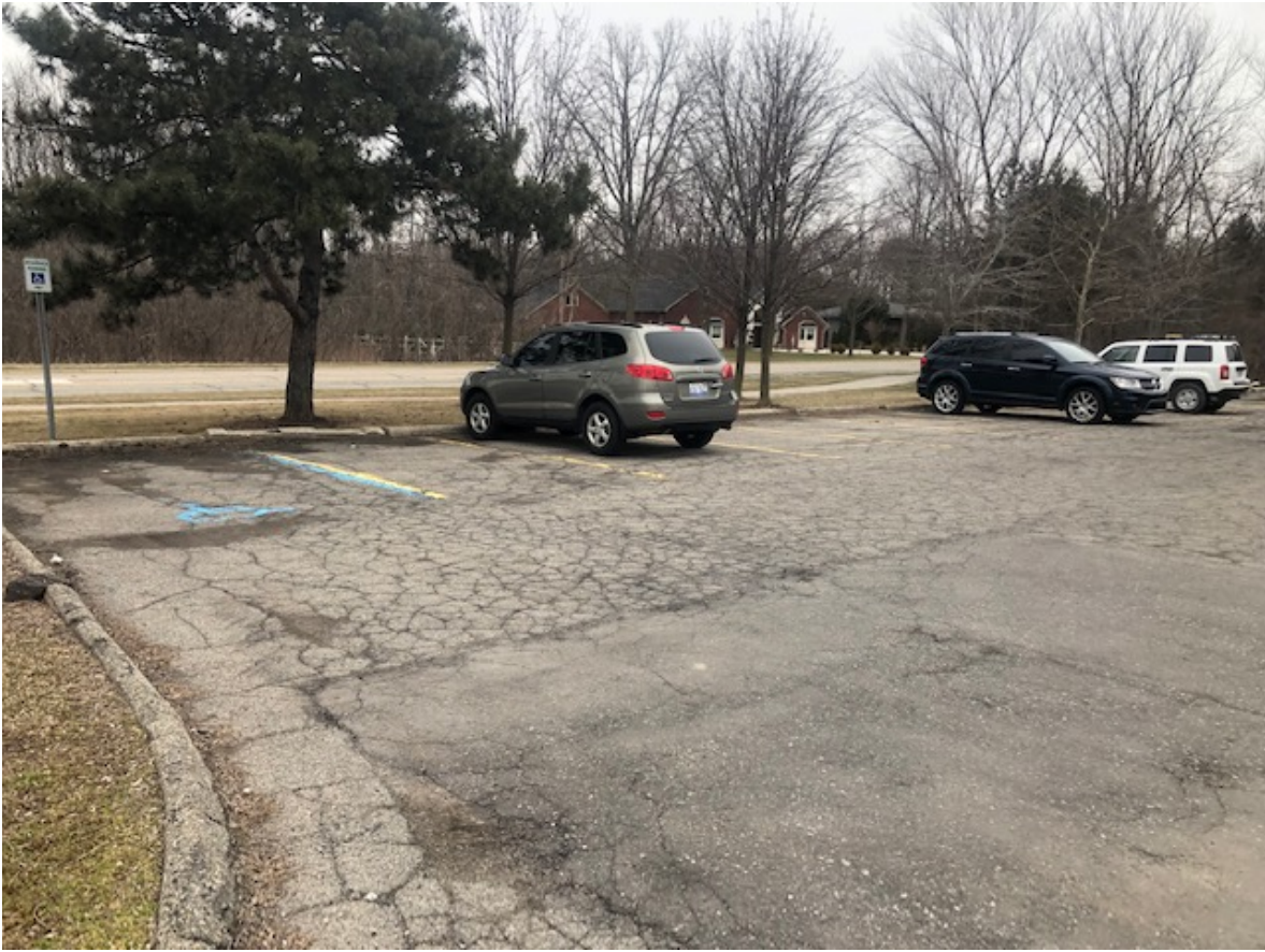
Before - Looking toward 11 Mile Road
