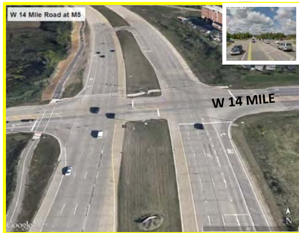
Figure 34. M5 at 14 Mile Road
