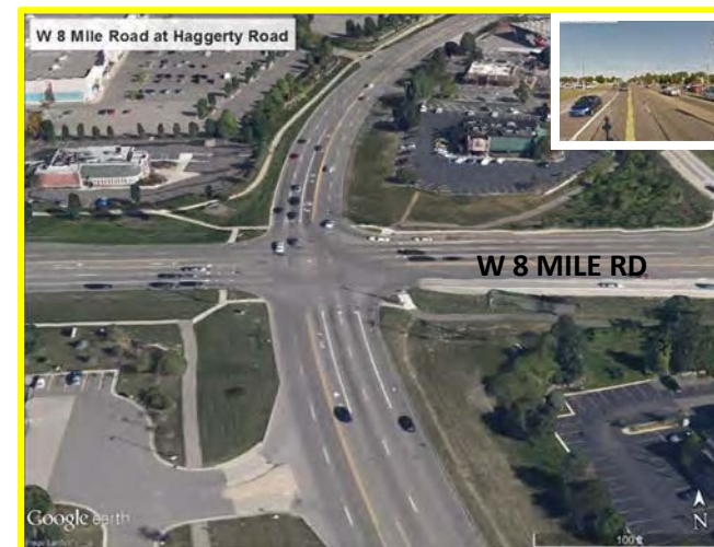
Figure 31. Haggerty Road at 8 Mile Road
