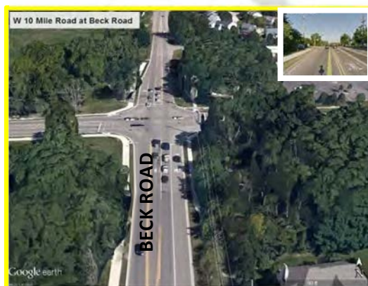
Figure 21. Beck Road at 10 Mile Road
