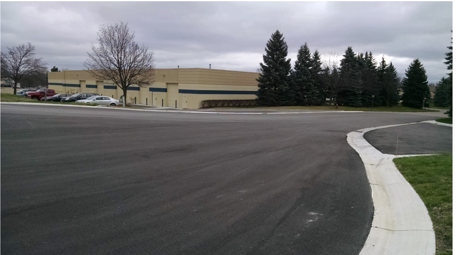
West-side of cul-de-sac, looking east
