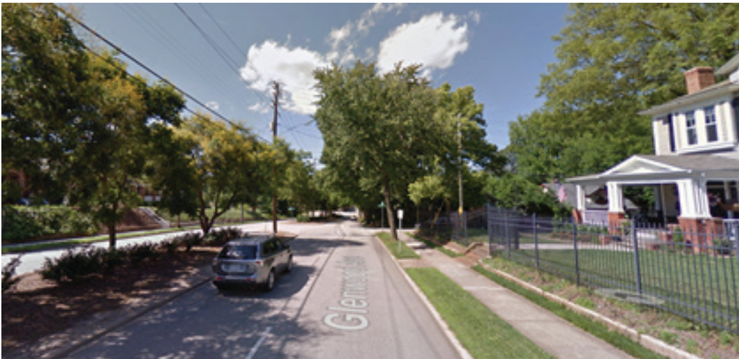
A particular problem facing older neighborhoods occurs when a thoroughfare fronted by older homes is widened to four or more lanes, threatening the fronting homes and neighborhoods with decline. The impact of such widenings on homes can be mitigated through a variety of means, including retrofitting the road with a median, skinnying lanes, retrofitting front yards with low fences or walls, creating front yard grade elevations above road level, and others. Some towns also consider rezoning the fronting properties to allow redevelopment with townhomes, patio homes, or small multifamily.
