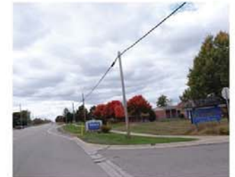
20 Lack of a significant identity and gateway image
