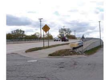
12 The bridge offers gateway opportunities and needs enhancement
