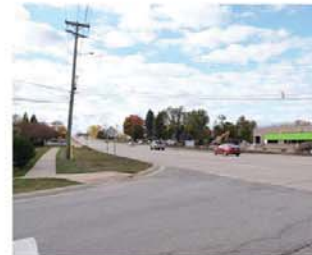
11 The corridor lacks amenities such as pedestrian lighting
