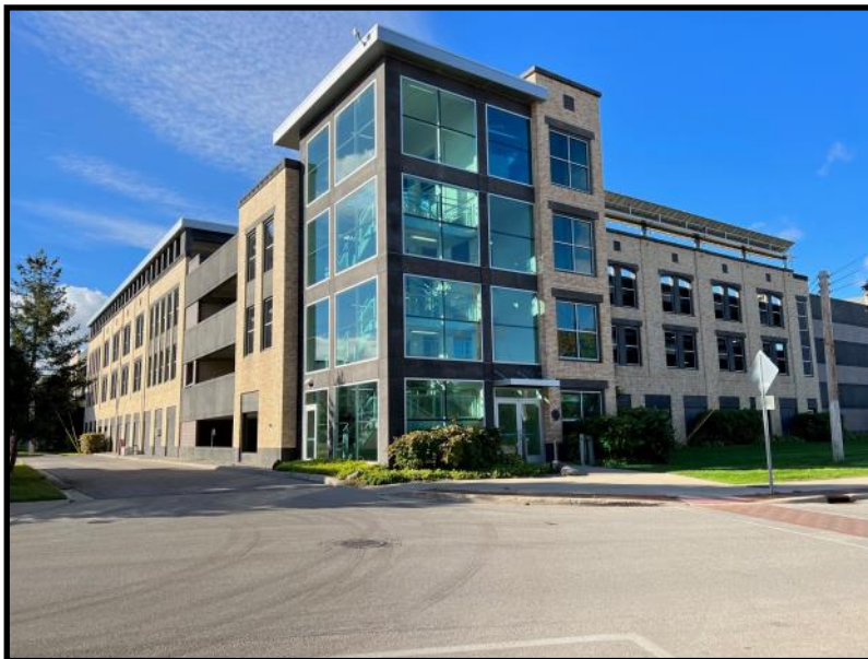
Figure E27: Parking structure in Traverse City
