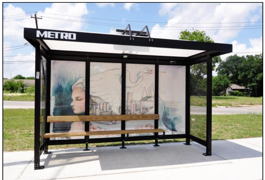
Figure C11: bus shelter in Houston, courtesy of ricedesignalliance.org
