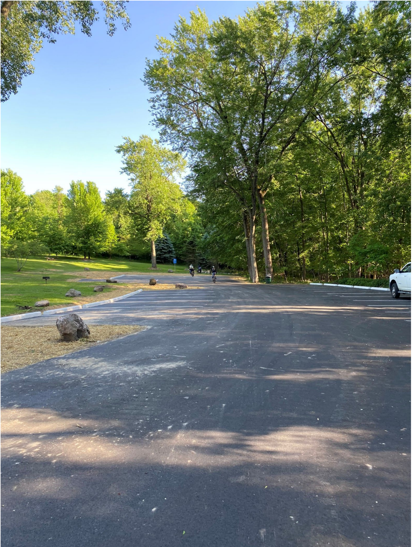
After – New south end of parking lot
