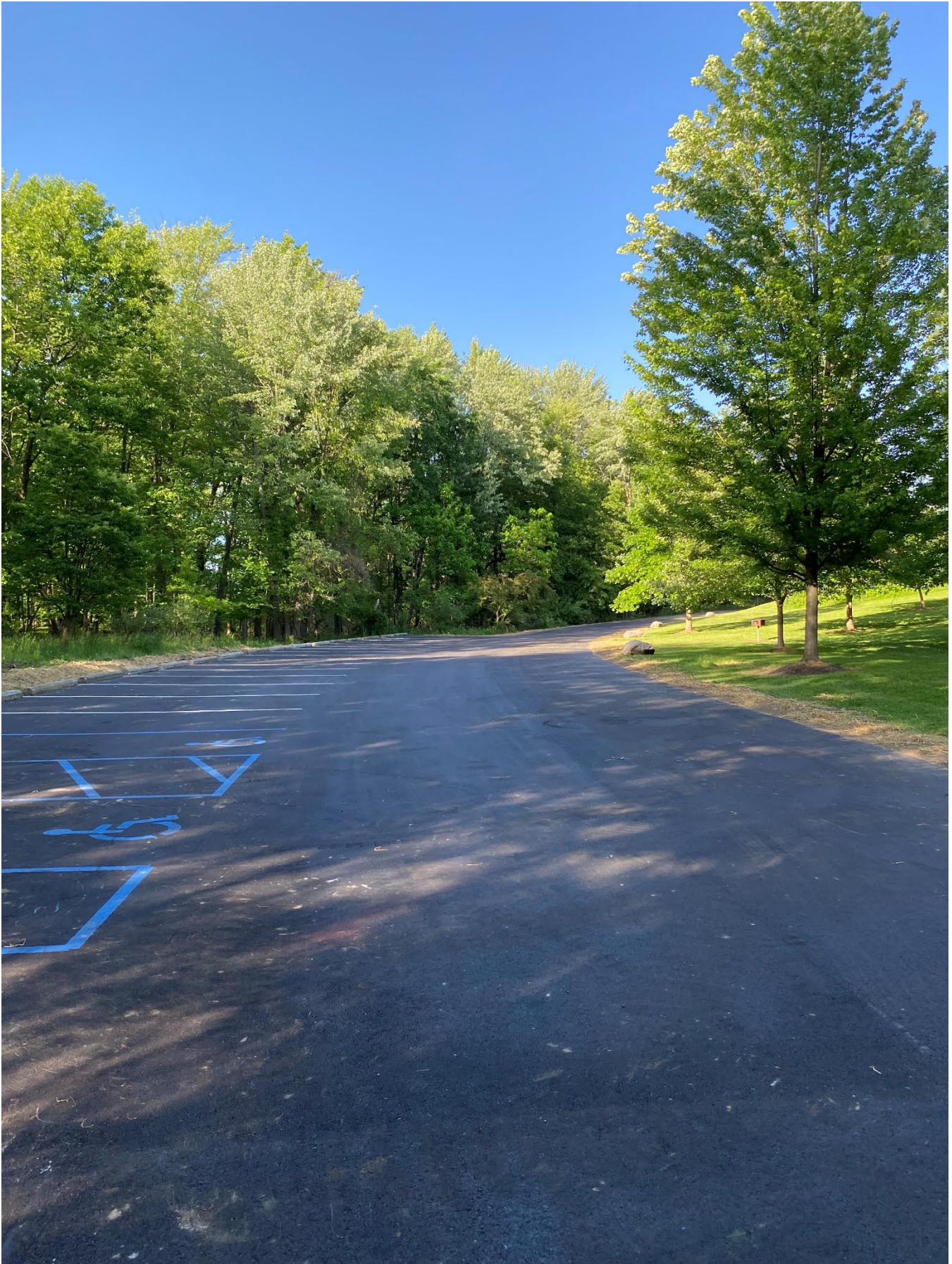
After – New north end of parking lot
