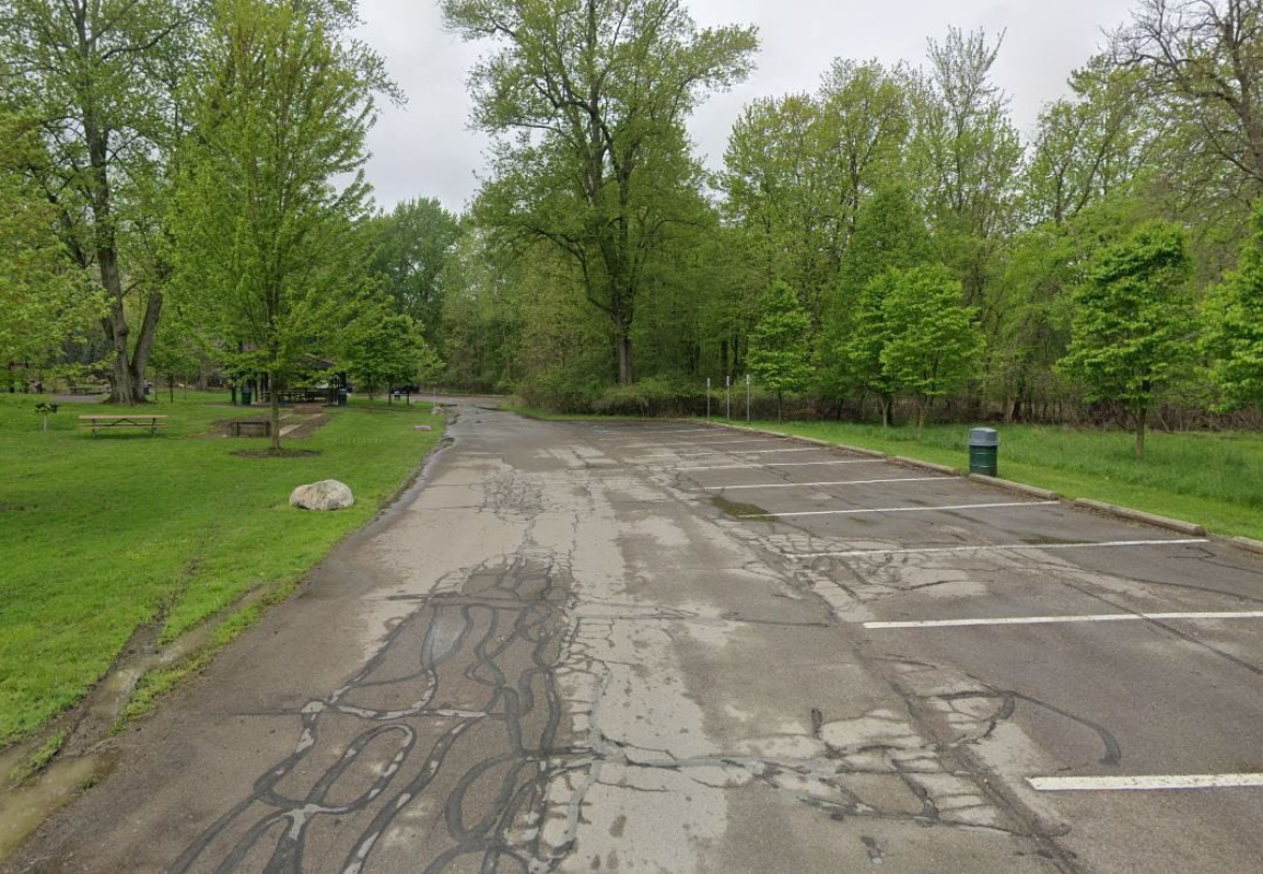
Before – Existing south end of parking lot, looking south
