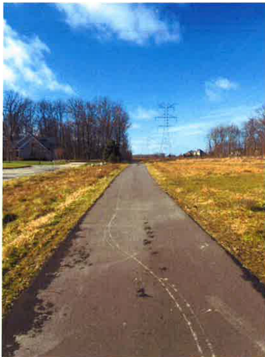
New 10-foot wide asphalt pathway along Deer Run, in the ITC Corridor.
