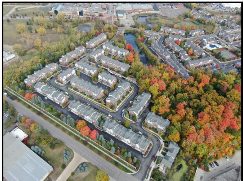
Figure D9: Main Street Village, pictured to the right, is an example of low-rise multi-family that could be built within a 200-foot buffer of single-family residential uses
