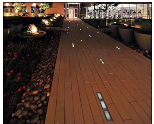
Figure E33: Solar-powered light-up paving in Dallas, TX; photo courtesy of Lea Stewart
