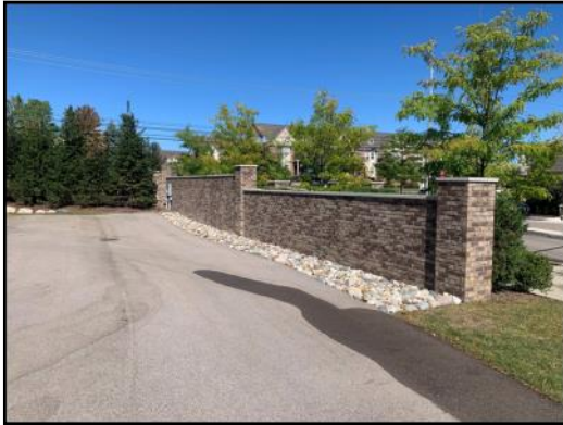
Figure E11: Huntley Manor Apartments in Novi has screening that separates Grand River, a major arterial, from residential units. Both decorative walls and landscaping in the form of trees were used to screen the homes from the street.
