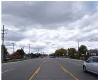
13 The width of pavement visually dominates the scale
