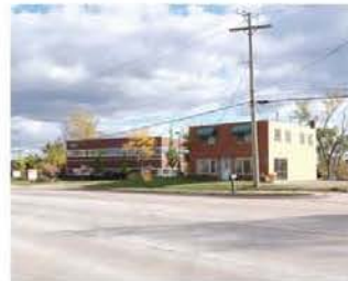
10 The corridor lacks unifying characteristics
