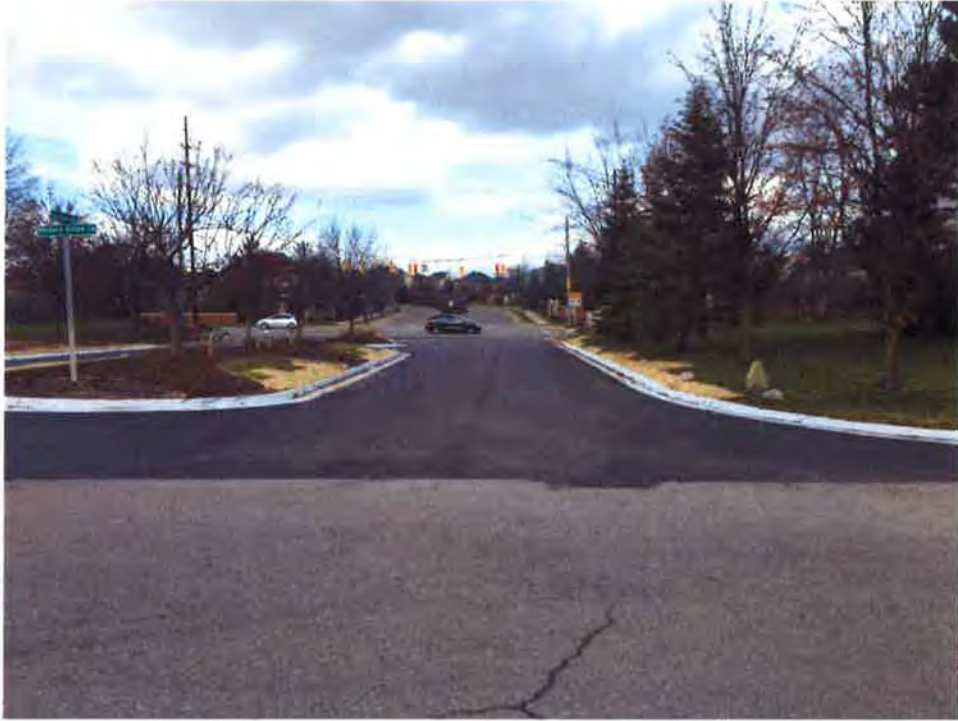
Exit Lane of Cortland Boulevard – Looking north towards 10 Mile Road
