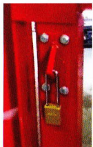
Combination and pad lock cutting.
