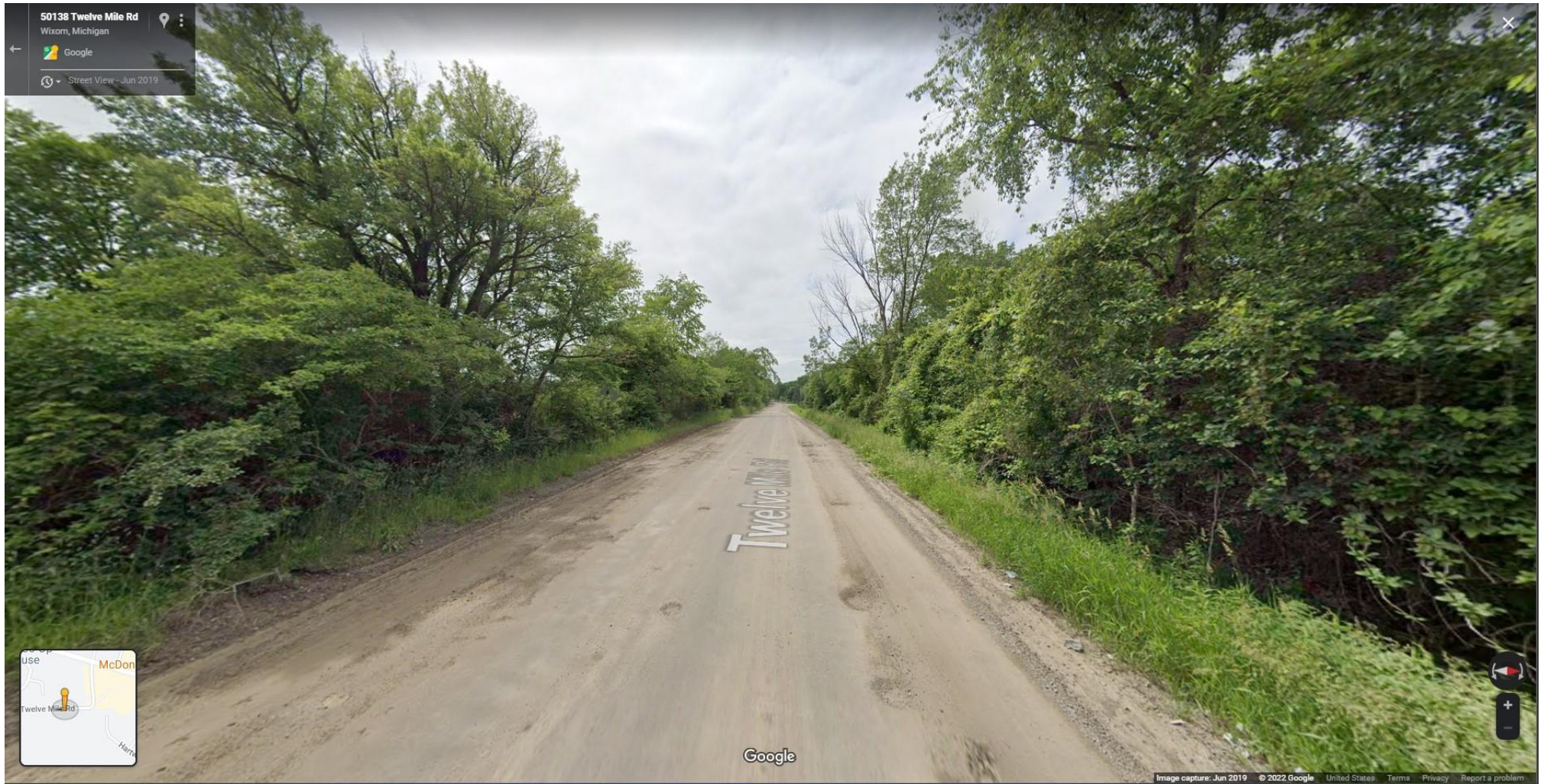
12 Mile Road, looking West
