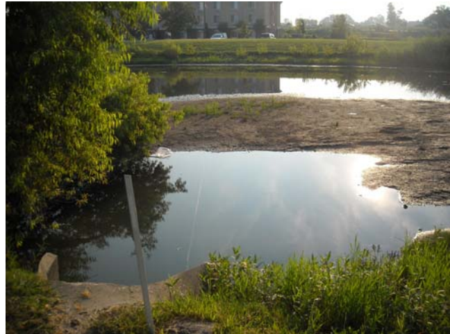
Sediment Accumulation at Basin #2
