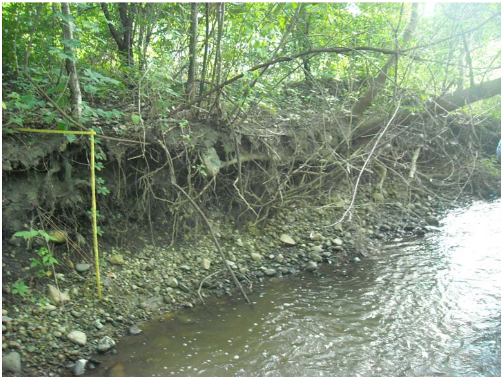
Undercutting Bank, looking downstream
