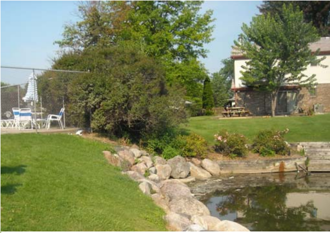
Village Oaks Lake Outlet Structure Hidden by Landscaping
