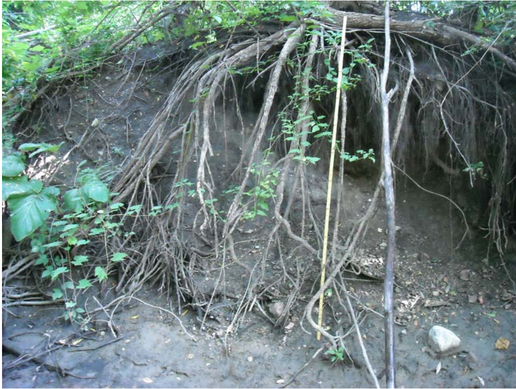
Undercutting Bank, Bank Height = ~ 7', BEHI = 29/Very High
