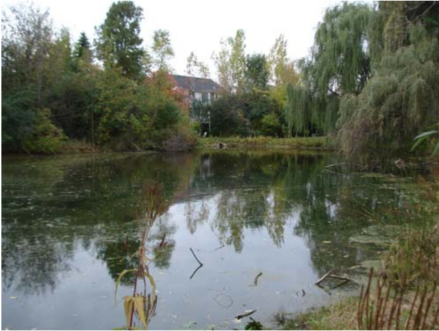
Lexington Green Detention Basin Outlet
