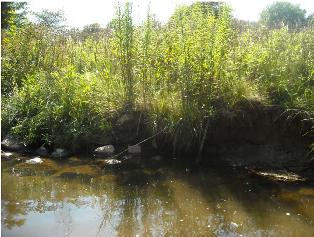
Active Bank Failure and Slumping
