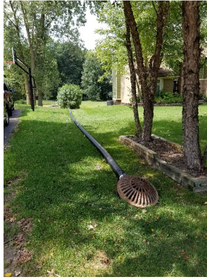
Piping along resident's yard
