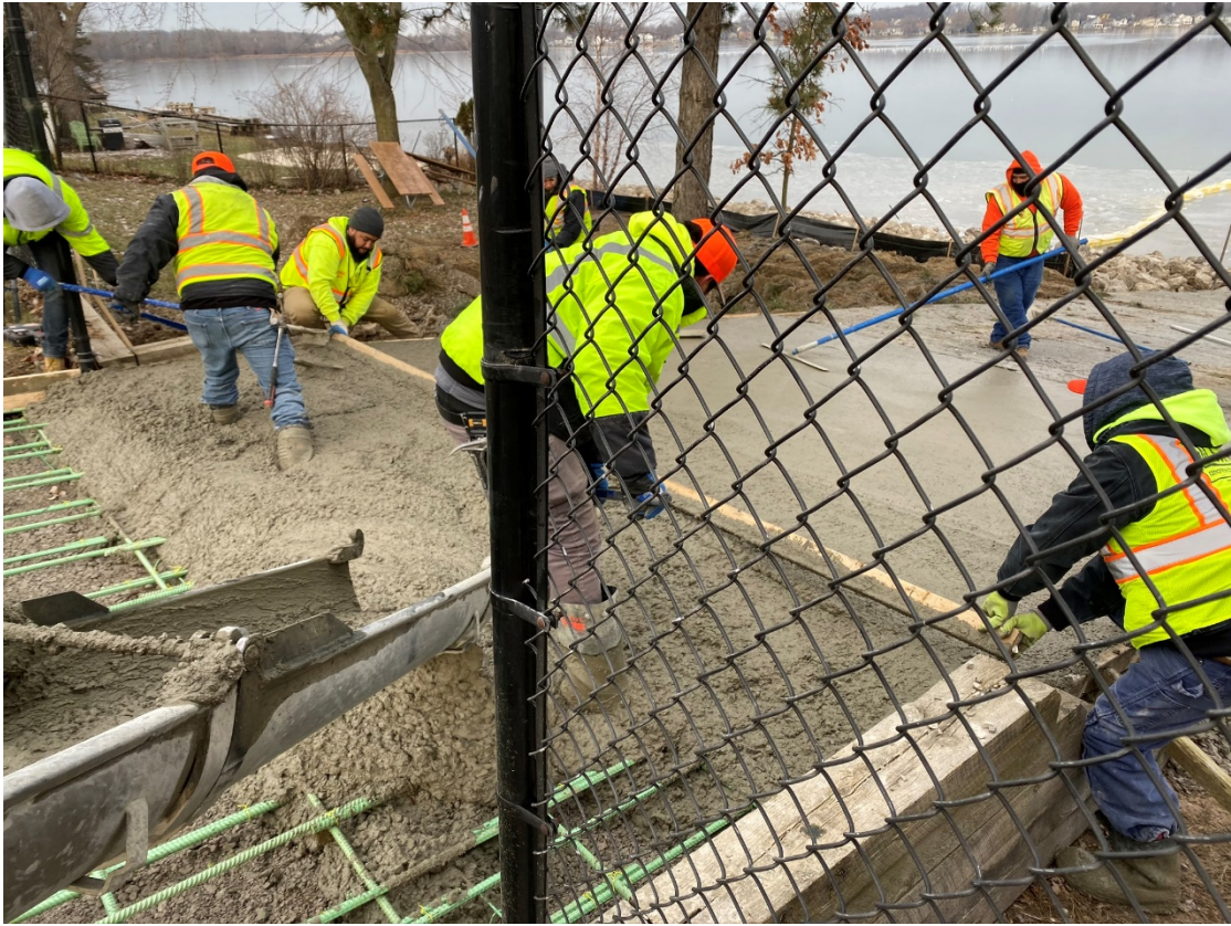
Lakeshore Park – concrete pour of the new boat launch.
