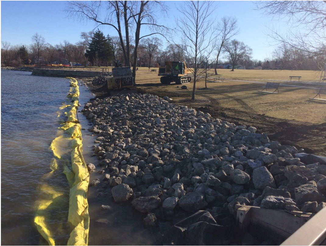
Pavilion Shore Park – Western rip-rapped shoreline near the wooden boardwalk look-out.
