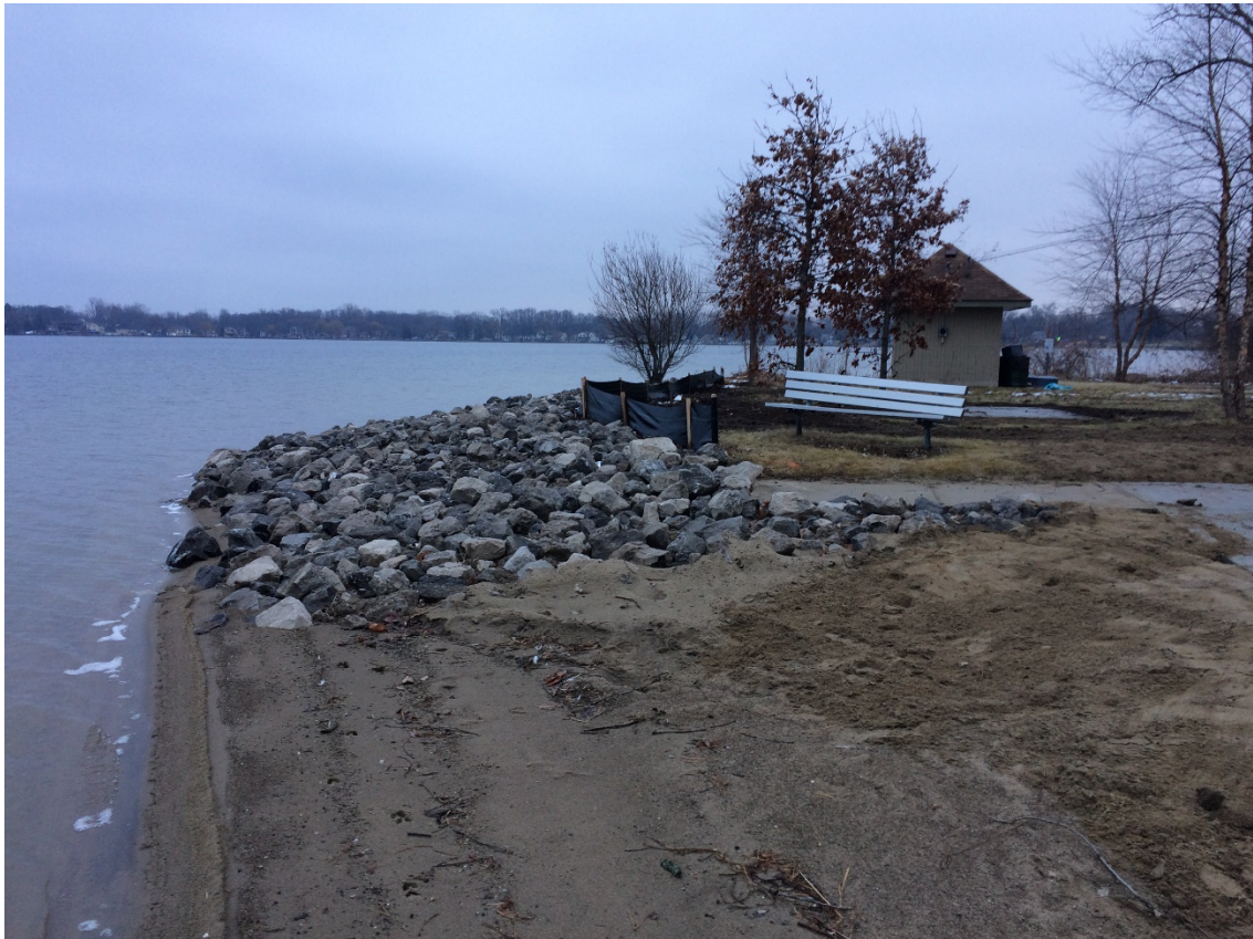
Lakeshore Park – Eastern rip-rap anchored shoreline stabilization
