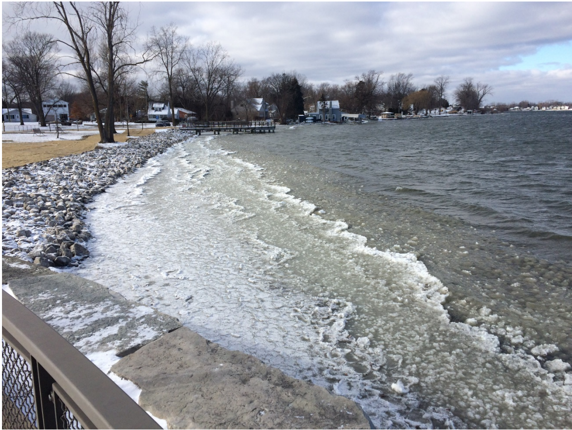
Pavilion Shore Park – The winter after installation holding up well to the ice-floe.
