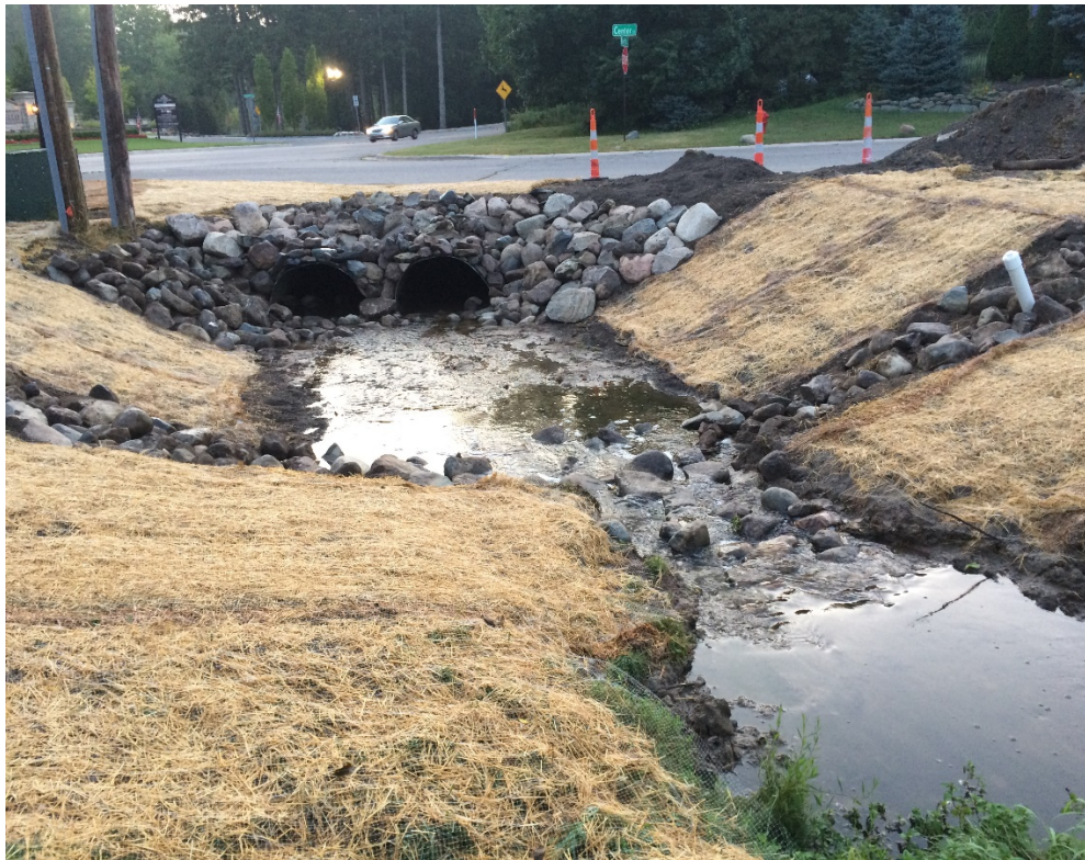
Thornton Creek – Restoration Complete.
