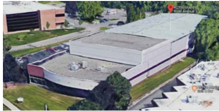
7 Existing Aerial - S.E. Corner SCALE: NTS REF:
