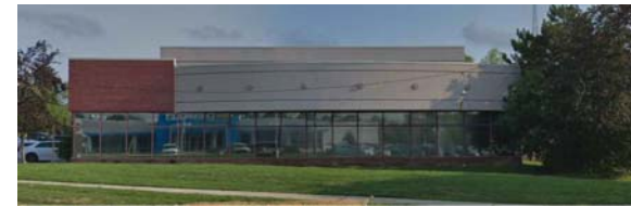
3 Existing Photo - South Elevation SCALE: NTS REF:
