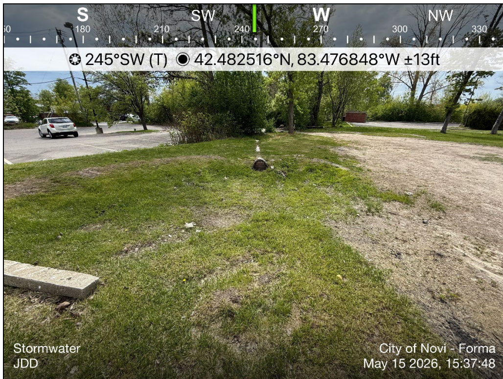
Overview of the stormwater pipe/area on-site
