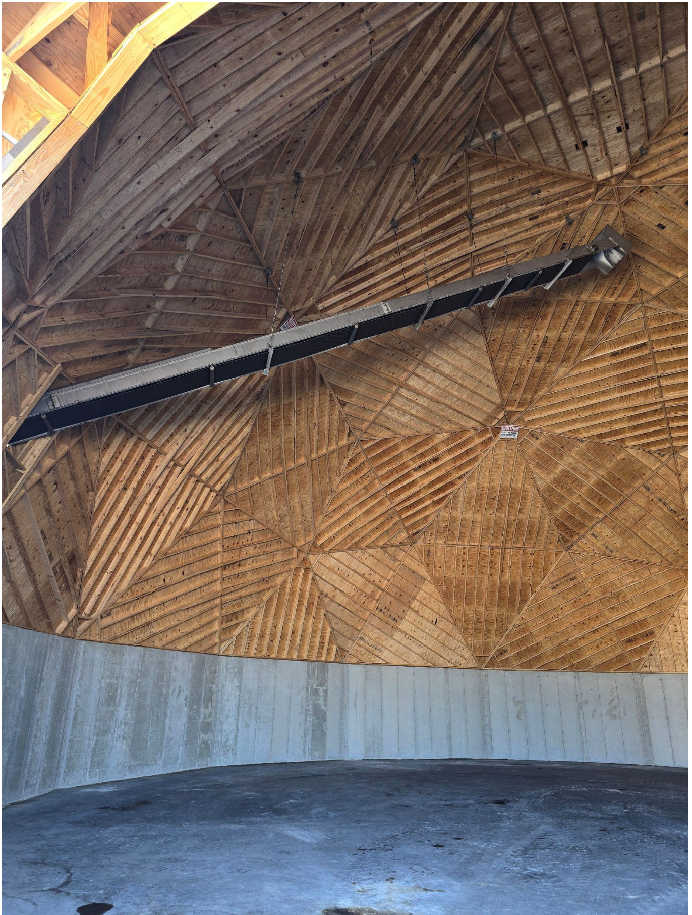
Interior view of the new concrete walls, conveyor, and roofing panels
