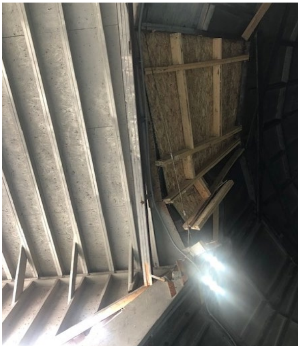
Pannel Damage and Temporary Repair
