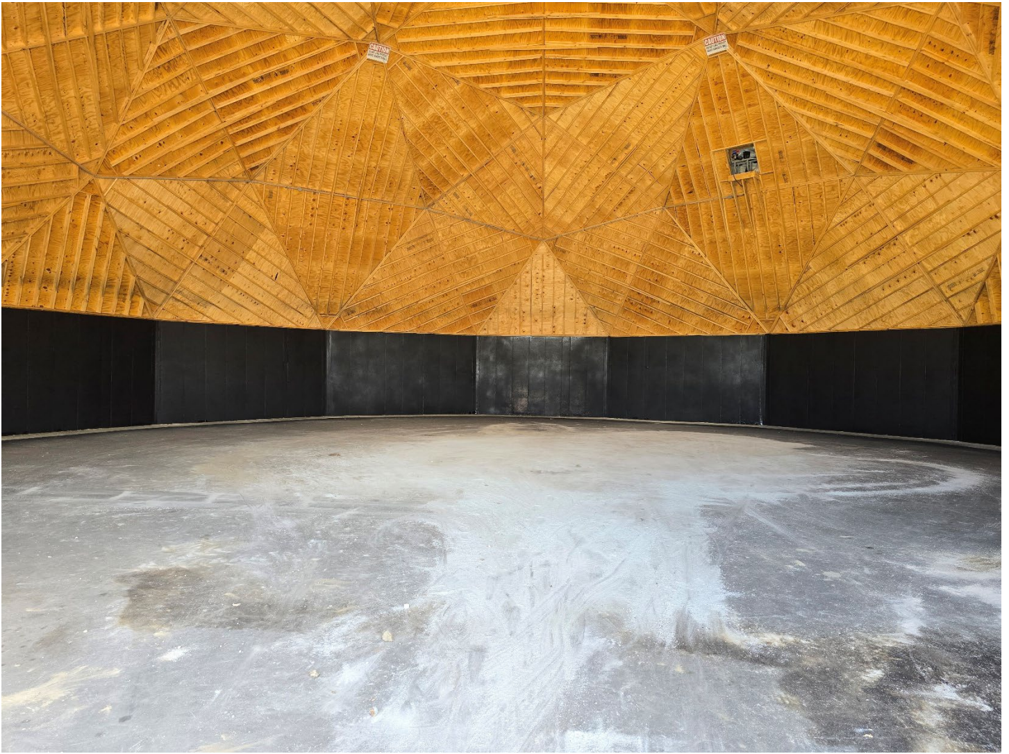
View of the concrete walls after applying a corrosion resistant liner
