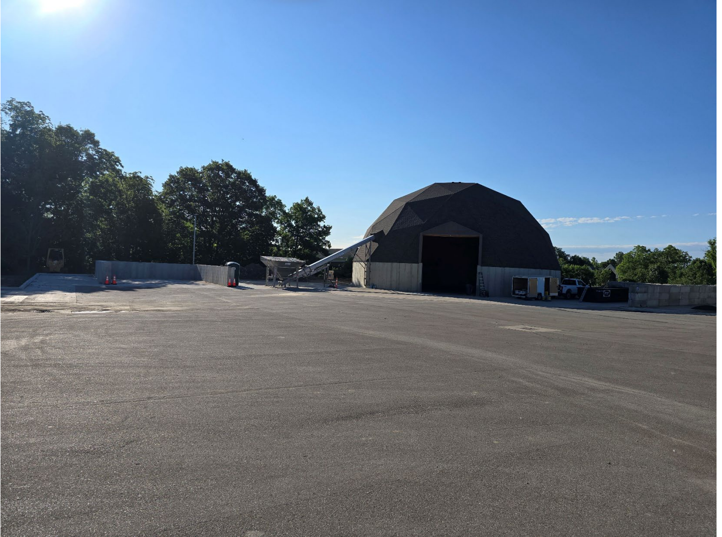
New, overall view of the salt dome, conveyor, and concrete storage bins
