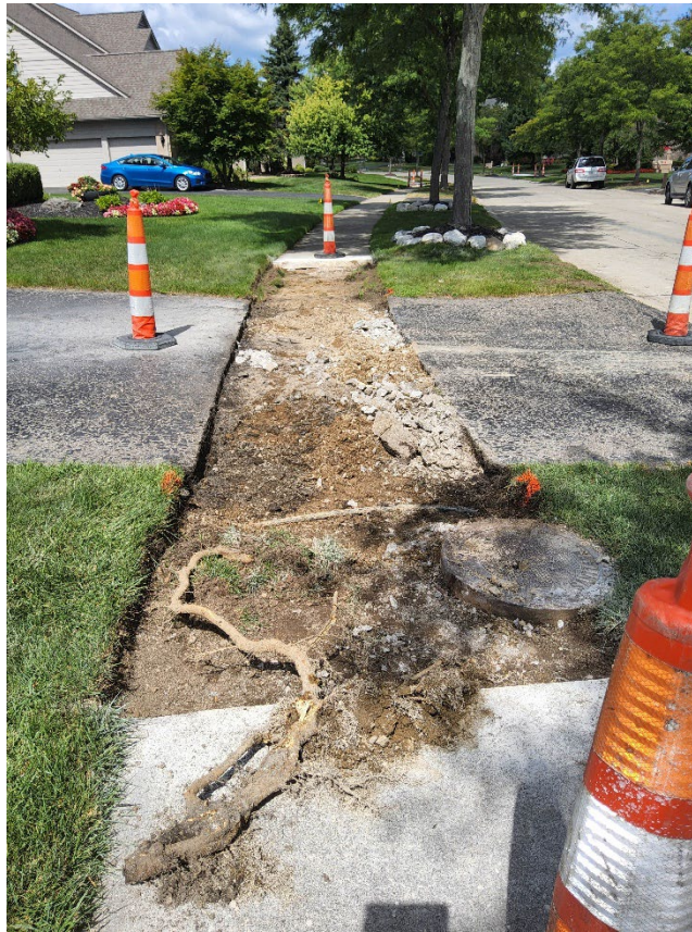
Before/During: 45593 Bristol Circle
