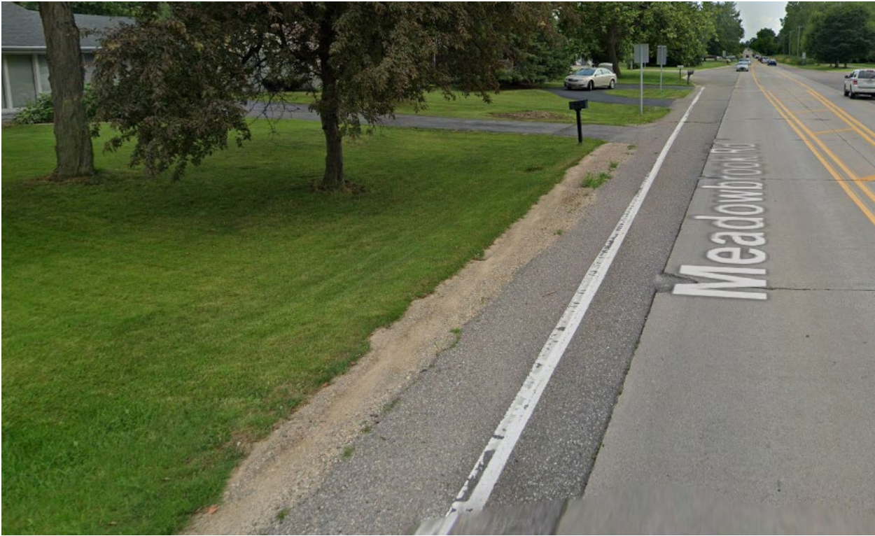
Example of an Enclosed Ditch on Meadowbrook Rd
