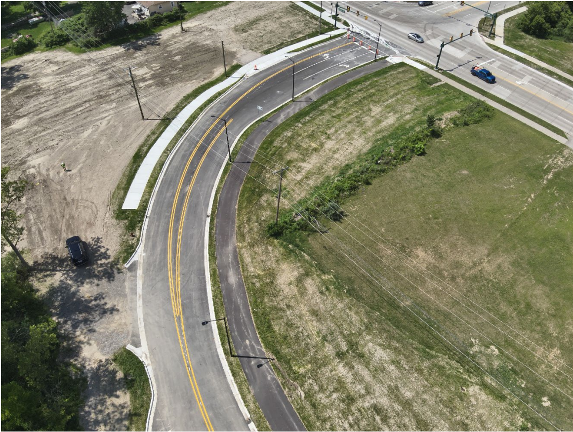
After – Aerial photo of Bond Street – Phase 2, looking northwest
