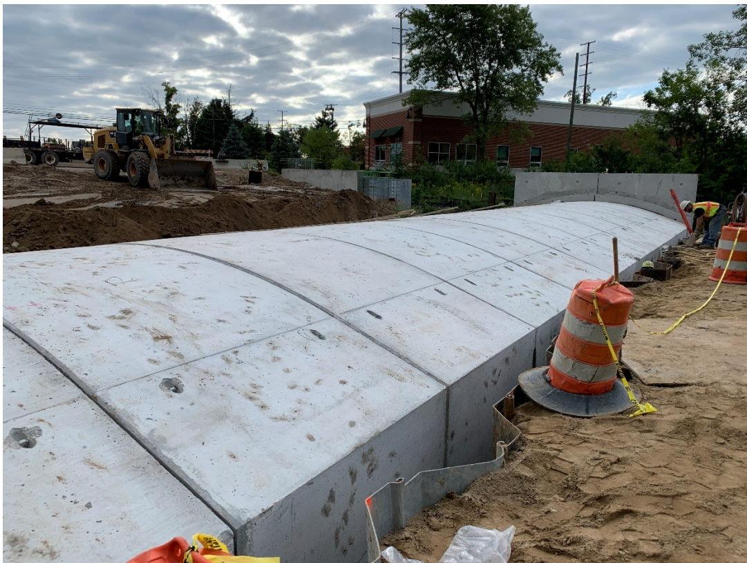
Completed box culvert over the Middle Rouge River.
