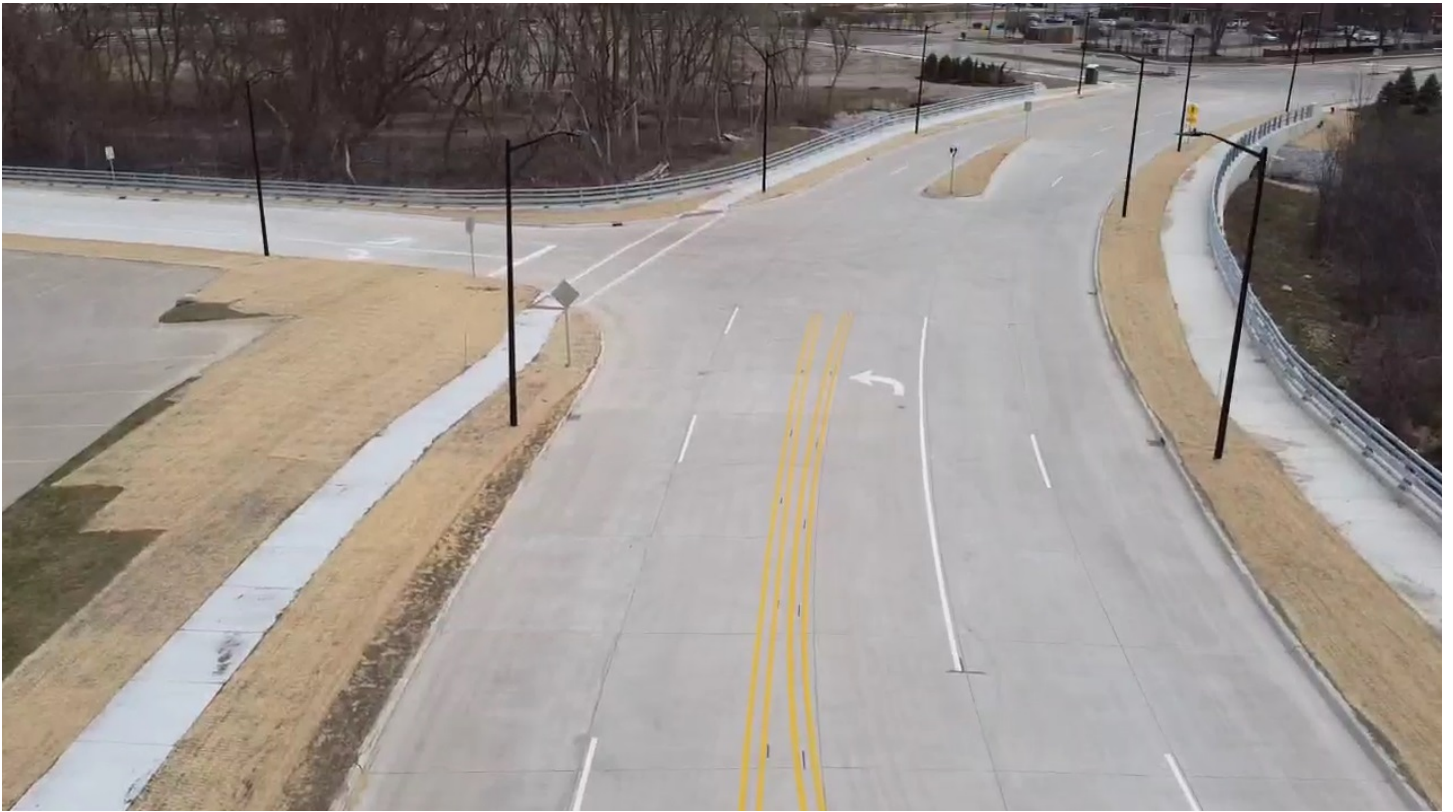
Open-to-Traffic at Industrial Spur (Lambert Drive) and new Crescent Boulevard.
