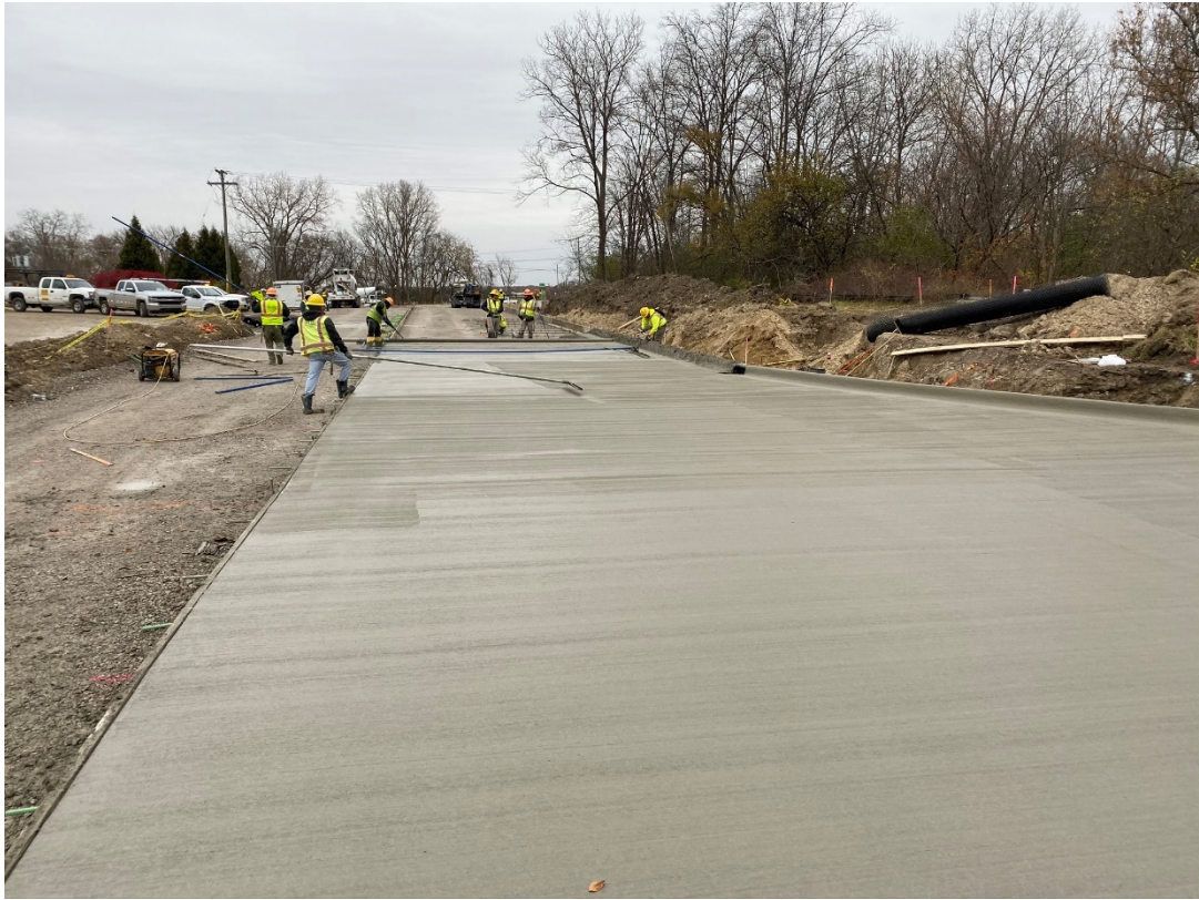
Pouring the northbound lanes of Crescent Boulevard from Grand River Avenue.
