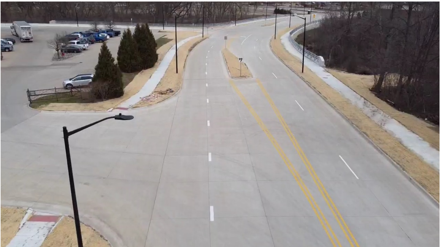
Open to Traffic at General Filters drive, looking north.
