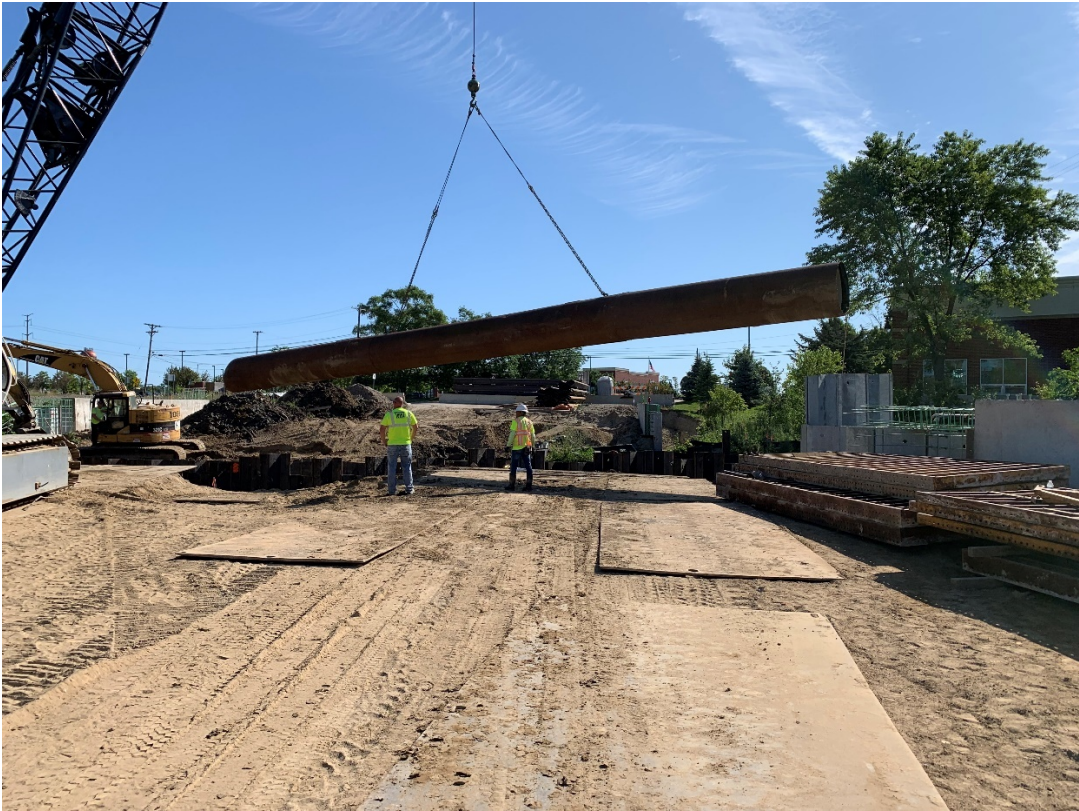
Installing temporary Middle Rouge River by-pass to construct new culvert.
