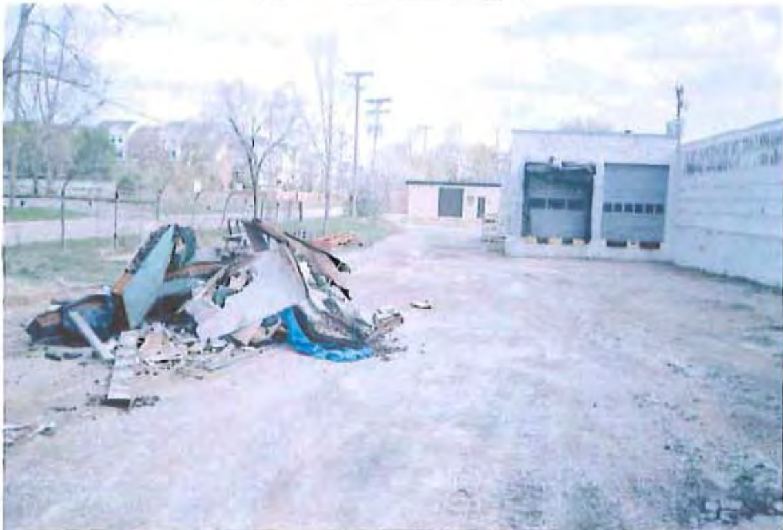
previous fence that was removed
