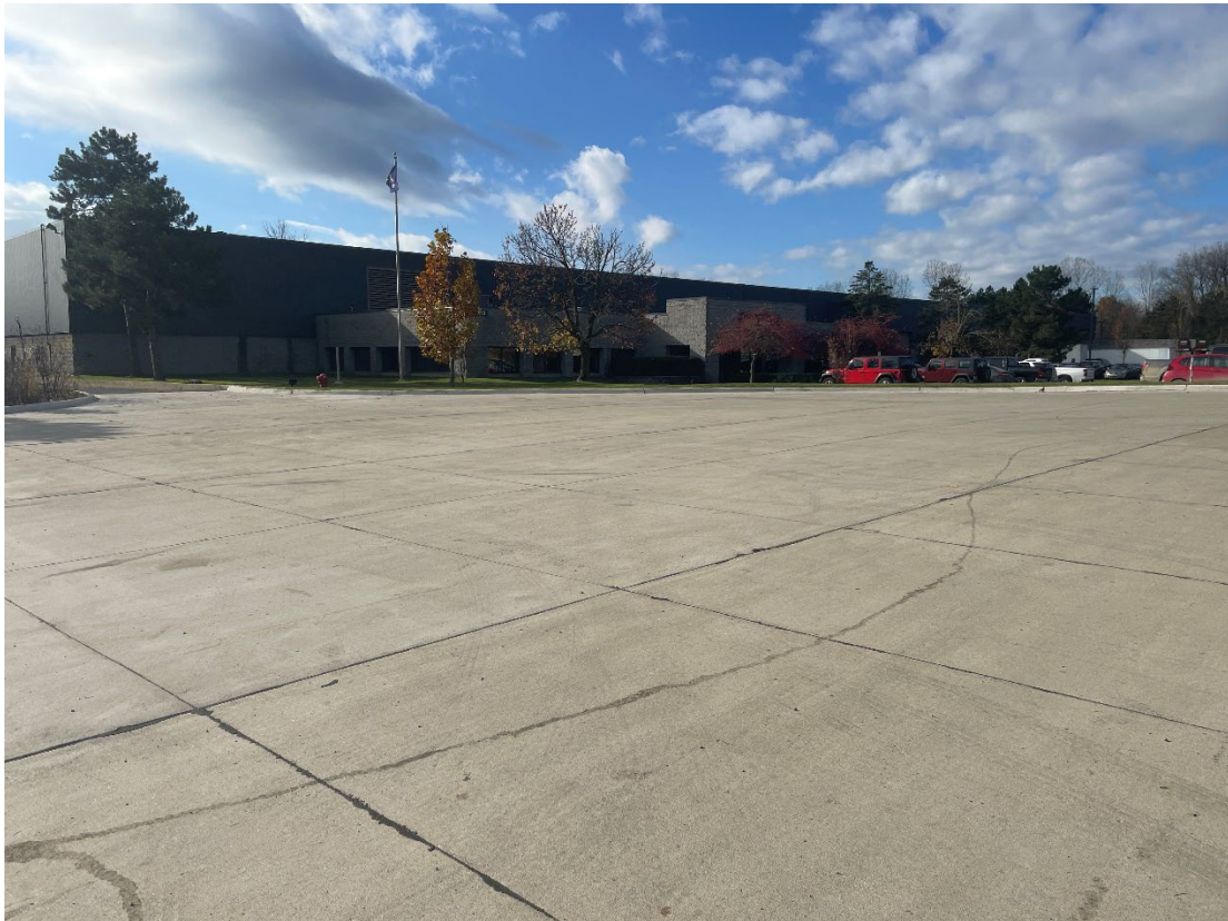
After – Gen-Mar Drive at cul-de-sac
