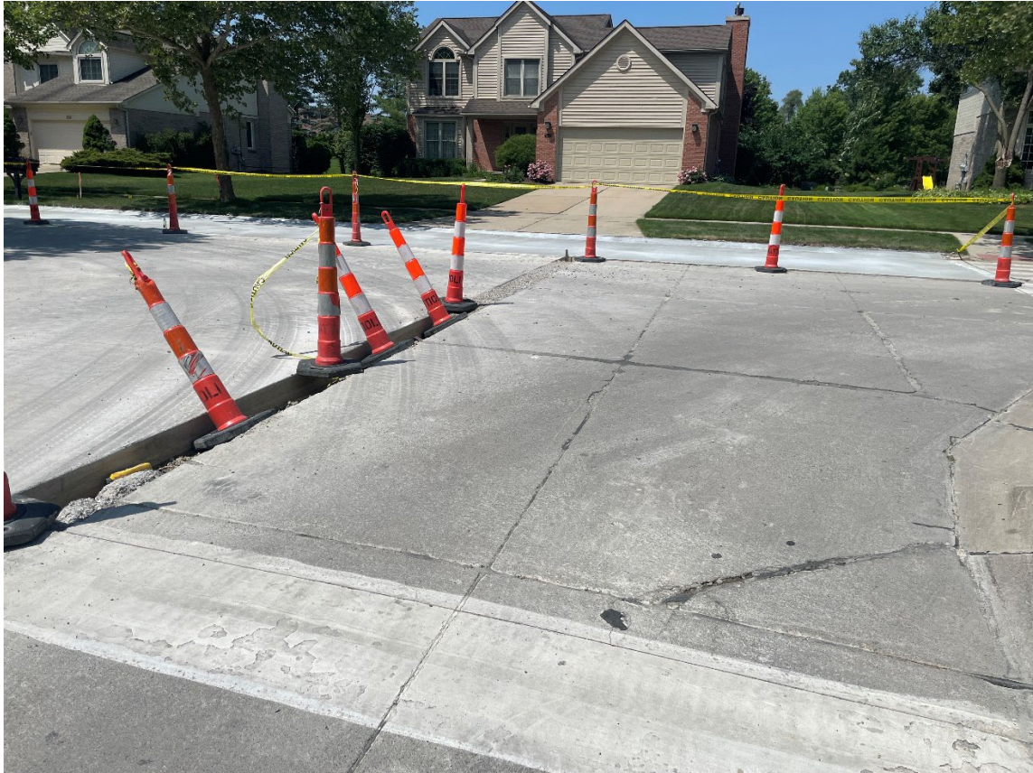
Before – Moorgate Street at Havergale Street
