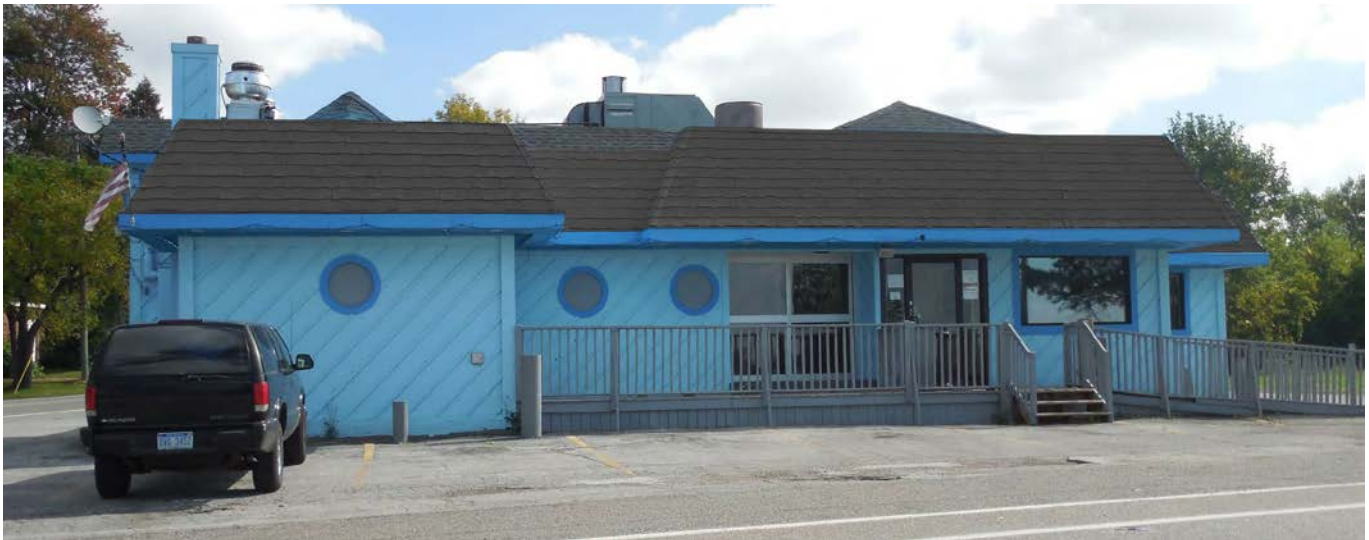
After as recommended with painting of asphalt shingles
