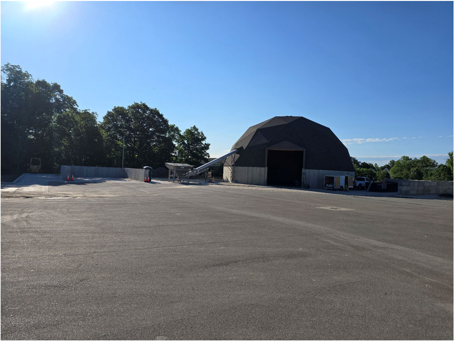
New Salt Dome, concrete bin/pit (left), and hopper/conveyor (7-18-25)
