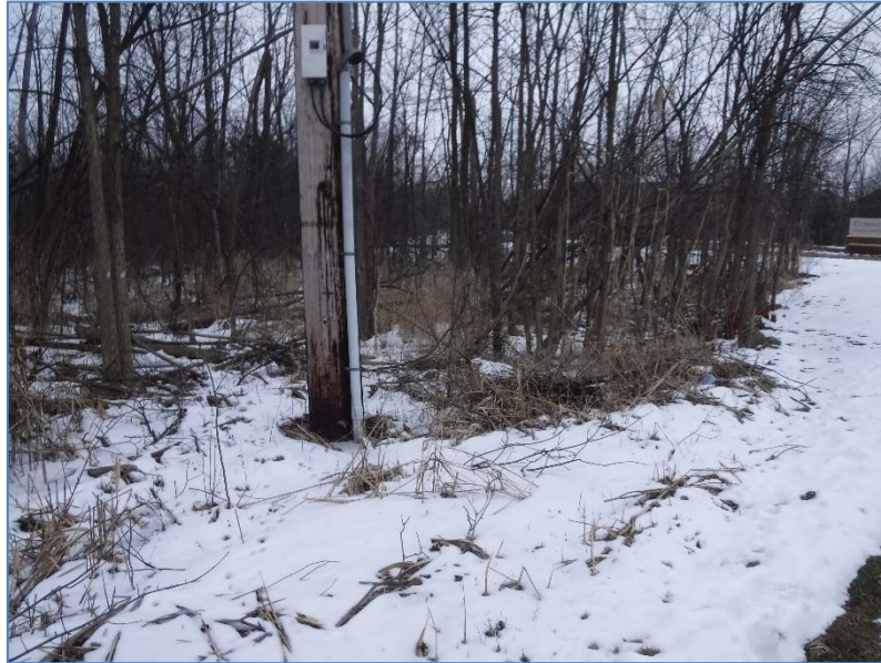
Photo 3. Looking north at the northern extents of the proposed project (ECT, January 31, 2020). Proposed area of impact to Wetland Area F as well as Regulated Woodland. This area is just south of the main entrance drive.
