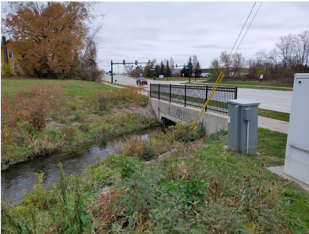
Figure 7. Northeast portion of AOI looking northwest, Walled Lake Branch in foreground.
