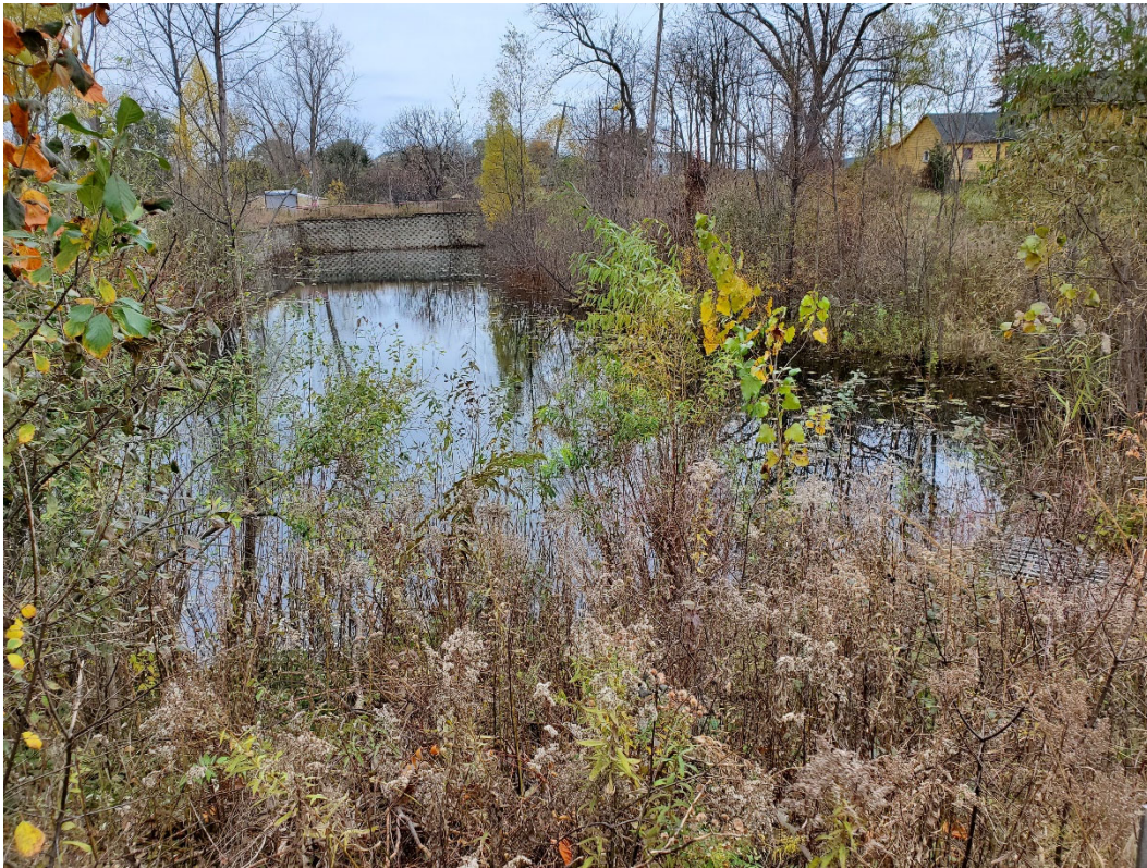
Figure 4. East side of the detention basin looking northwest.
