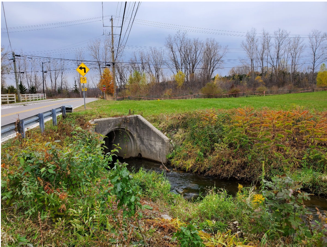
Figure 5. Northeast portion of AOI looking south, Walled Lake Branch in foreground.
