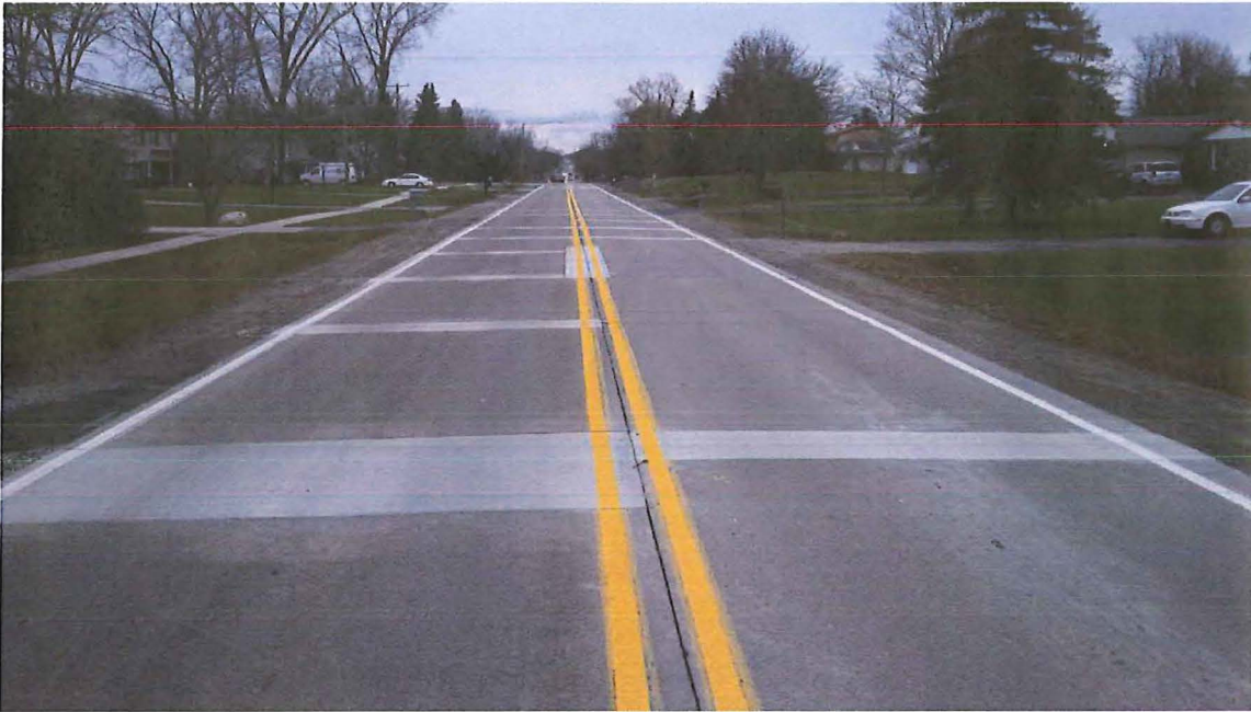
Looking north from Glyme Drive. Longitudinal and transverse joint replacements
