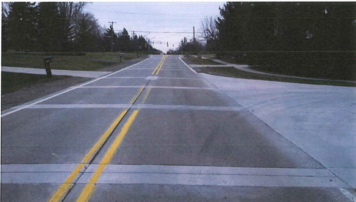
Looking south from Glyme Drive. Joint replacements and Glyme Dr. reconstruct
