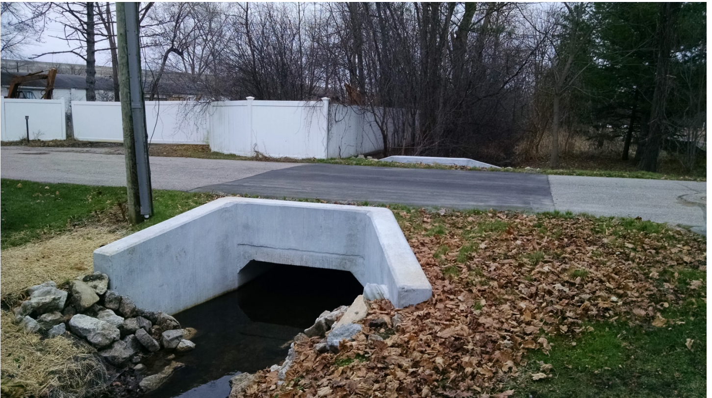
West side looking east along new culvert
