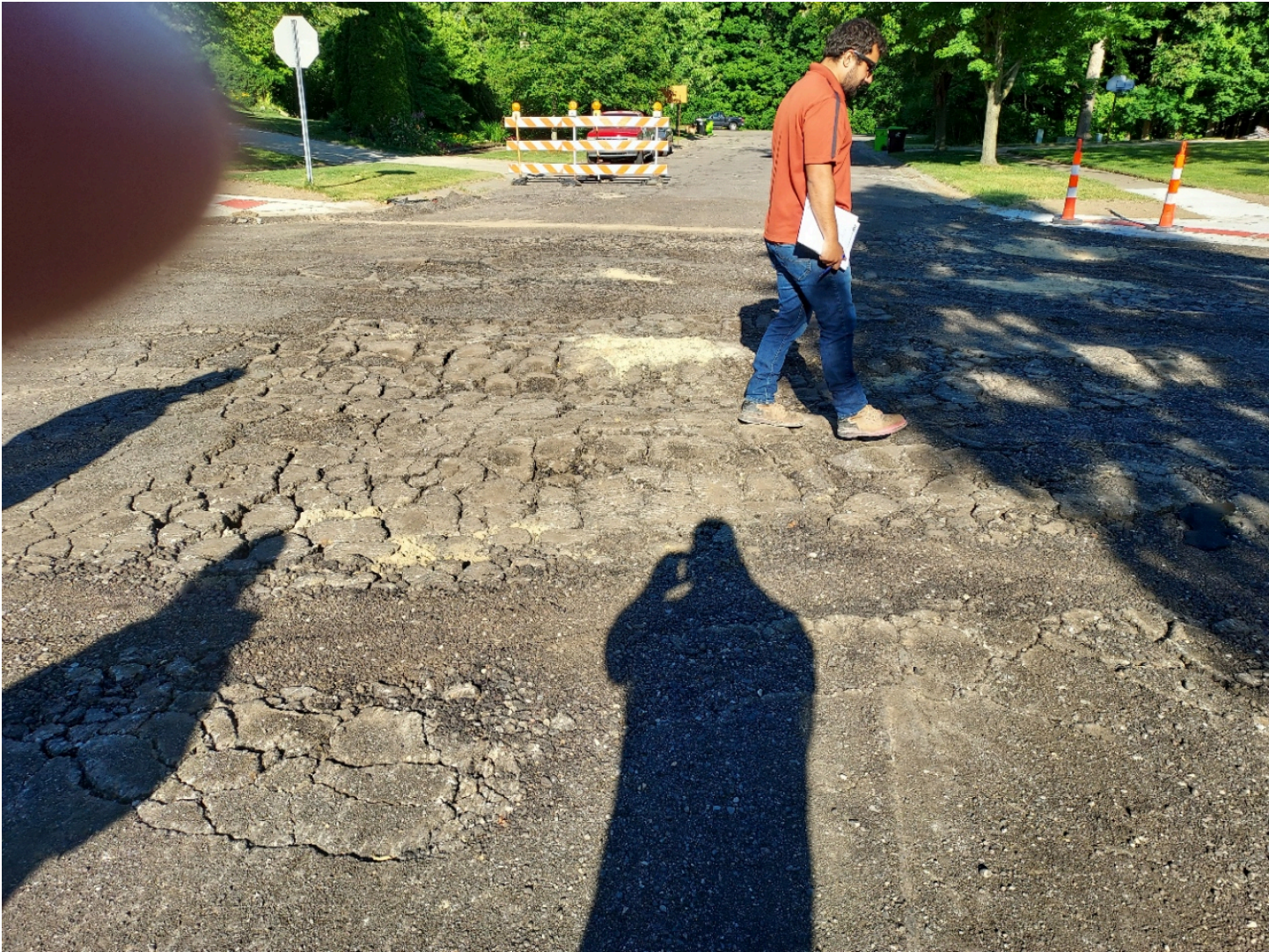
Looking east to west across Christina Lane, near Sussex Drive
