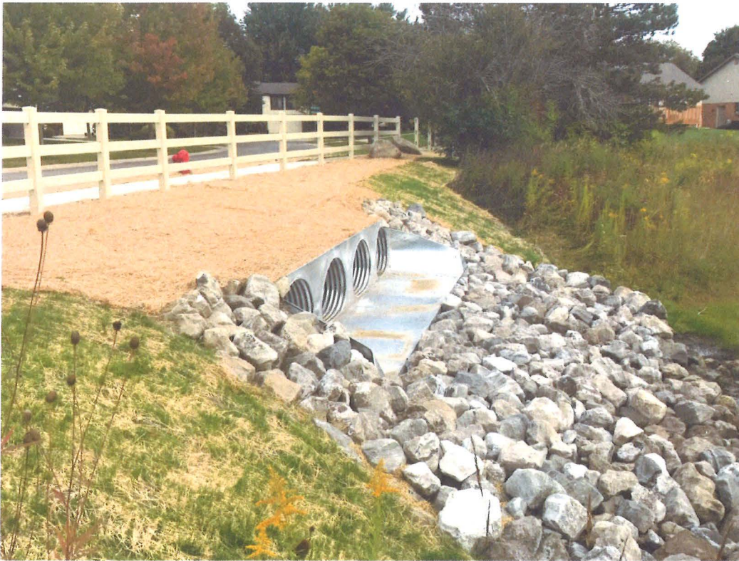
New one-piece headwall and elliptical culverts on east-side of Christina Lane.
