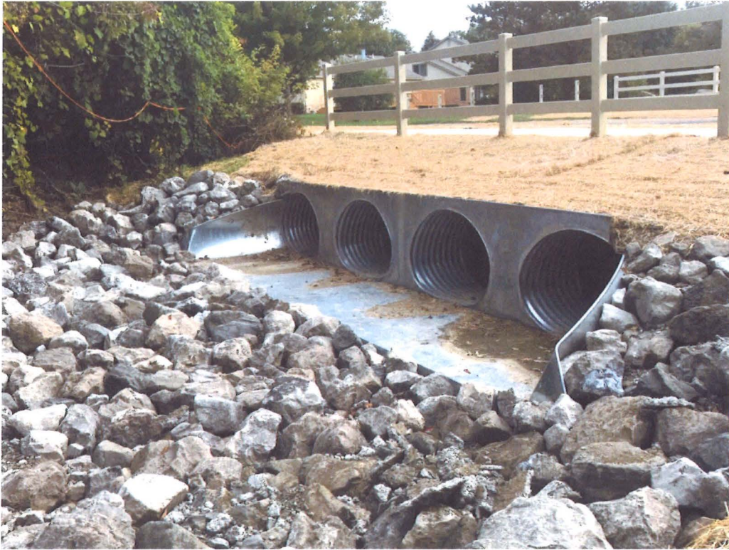
New one-piece headwall and elliptical culverts on west-side of Christina Lane.
