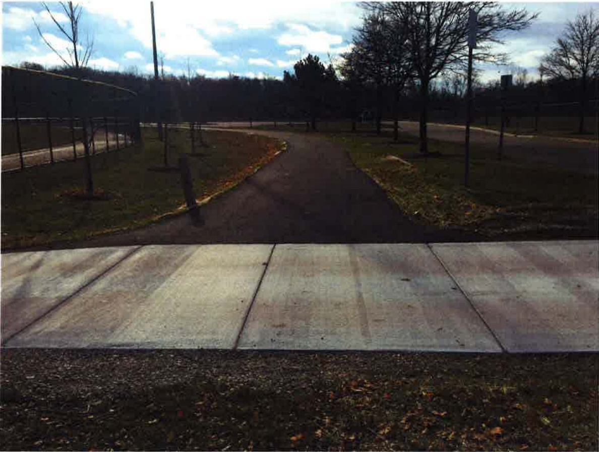
Replacement of asphalt/concrete paths in Power Park
