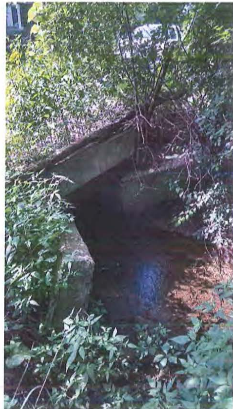
East End of Bridge
