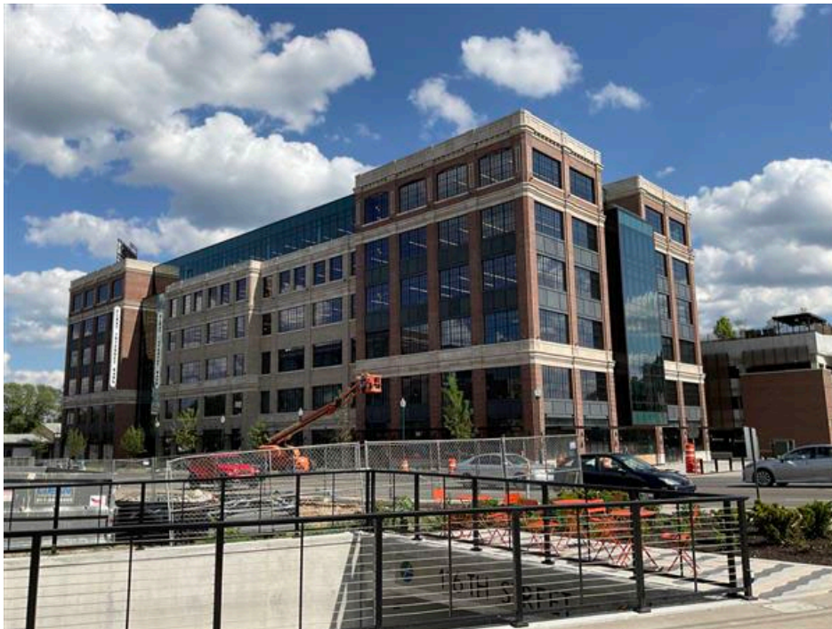
Large office/bank in the process of construction
