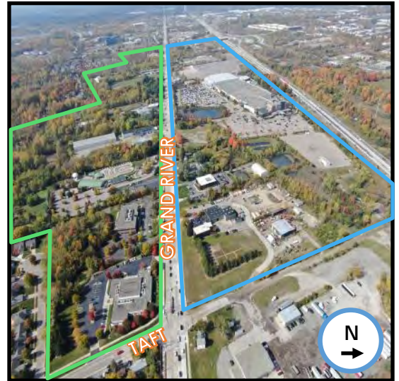
Figure B1 (below): Aerial of both City West areas
