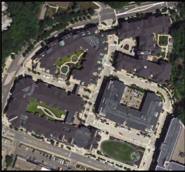
Figure D22: aerial of The Promenade in Wayzata, Minnesota
