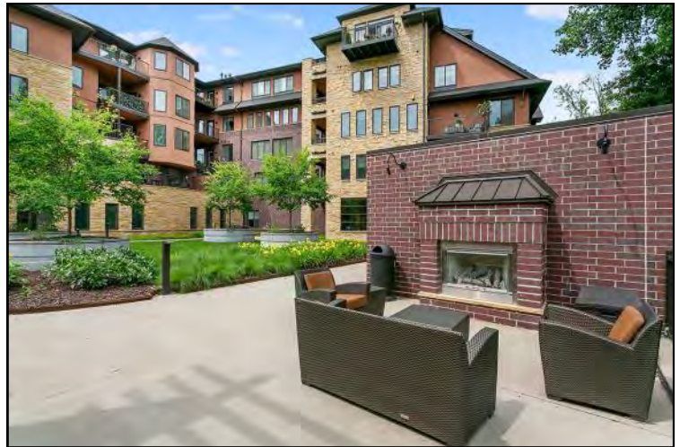
Figure D21: public seating and amenity a part of Folkestone, a senior residential community in Wayzata; source: preshomes.org
