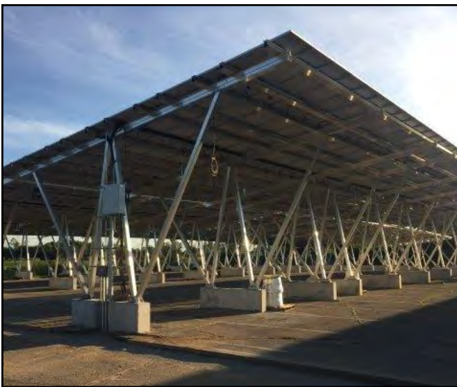
Figure D16: solar arrays built in parking lots on Michigan State University's campus
