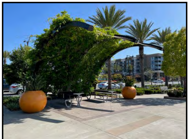
Figure D19: public seating and shade structure in San Diego, CA
