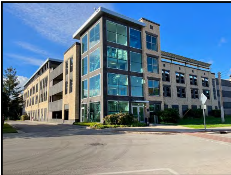
Figure E27: Parking structure in Traverse City
