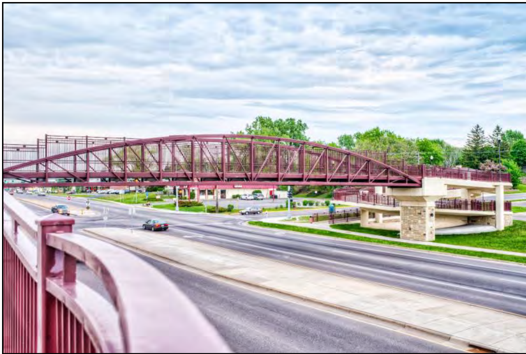
Figure C10: Pedestrian bridge with accessible switchback ramps in Columbia Heights, Minnesota. Photo courtesy of C.S. McCrossan
