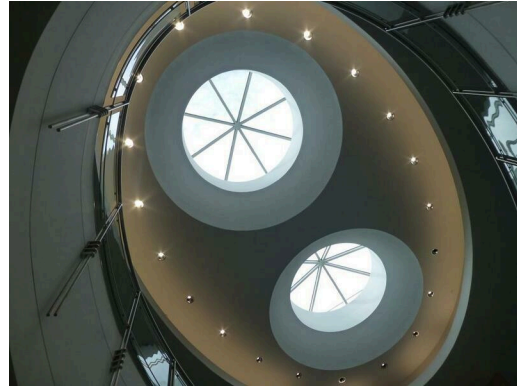
Skylights with LED Lights
