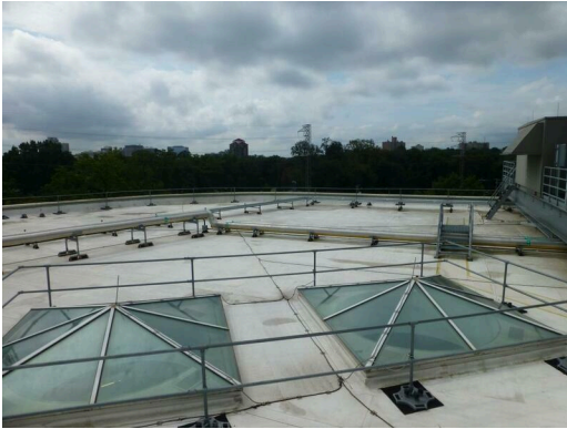
Rooftop at Bldg XXXX
